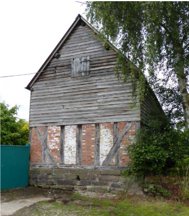
The gable end of a late 17th-century cow house to the north of Beeston, set on a stone plinth and with straight wall-bracing typical of this period. Photo © Jeremy Lake
