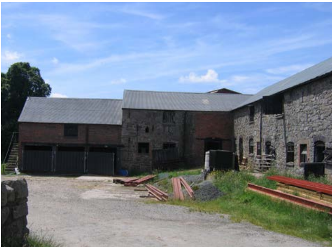
This L-shaped range in the lowlands comprises cattle housing to the right. At the junction between the two ranges is brick walling to a former threshing bay – with a stable on its left and, further to the left, a brick-built cart shed or granary range. Photo © Jeremy Lake
