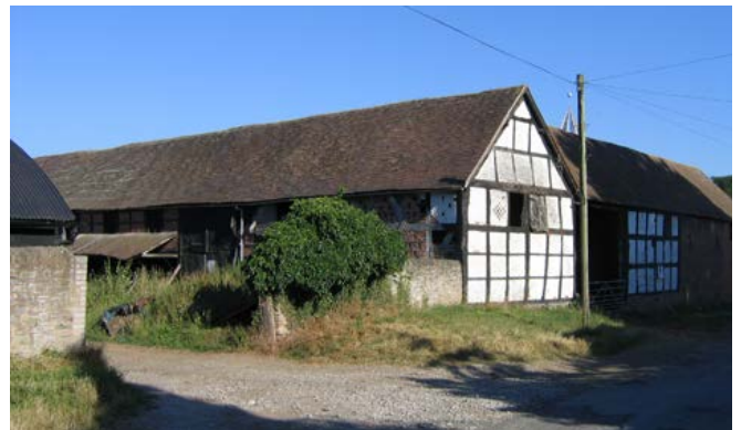
The largest timber-framed barns are concentrated in the arable west of the area. This has been extended into an L-plan – a common form. Photo © Bob Edwards
