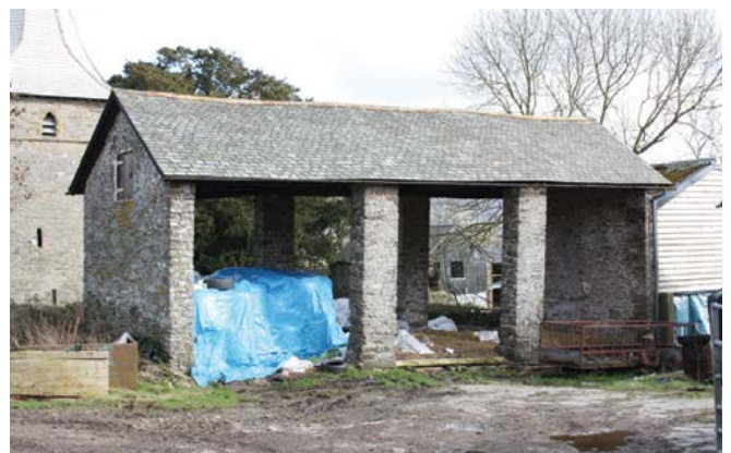
Open-sided, stone-built hay barns are found in small numbers, especially on larger farms across the lower lying parts of the area. Photo © Bob Edwards
