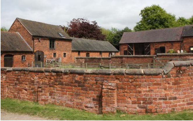
This farmstead originated as a loose courtyard plan. Over time buildings have been added to create long ranges to two sides of the yard, although the ranges remained detached from each other. Photo © Bob Edwards
