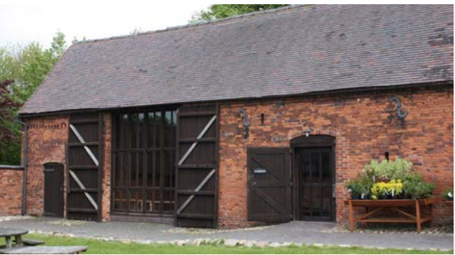
Brick-built barns feature on most farmsteads in this area. This barn is of four bays but barns of five bays are common. Photo © Bob Edwards
