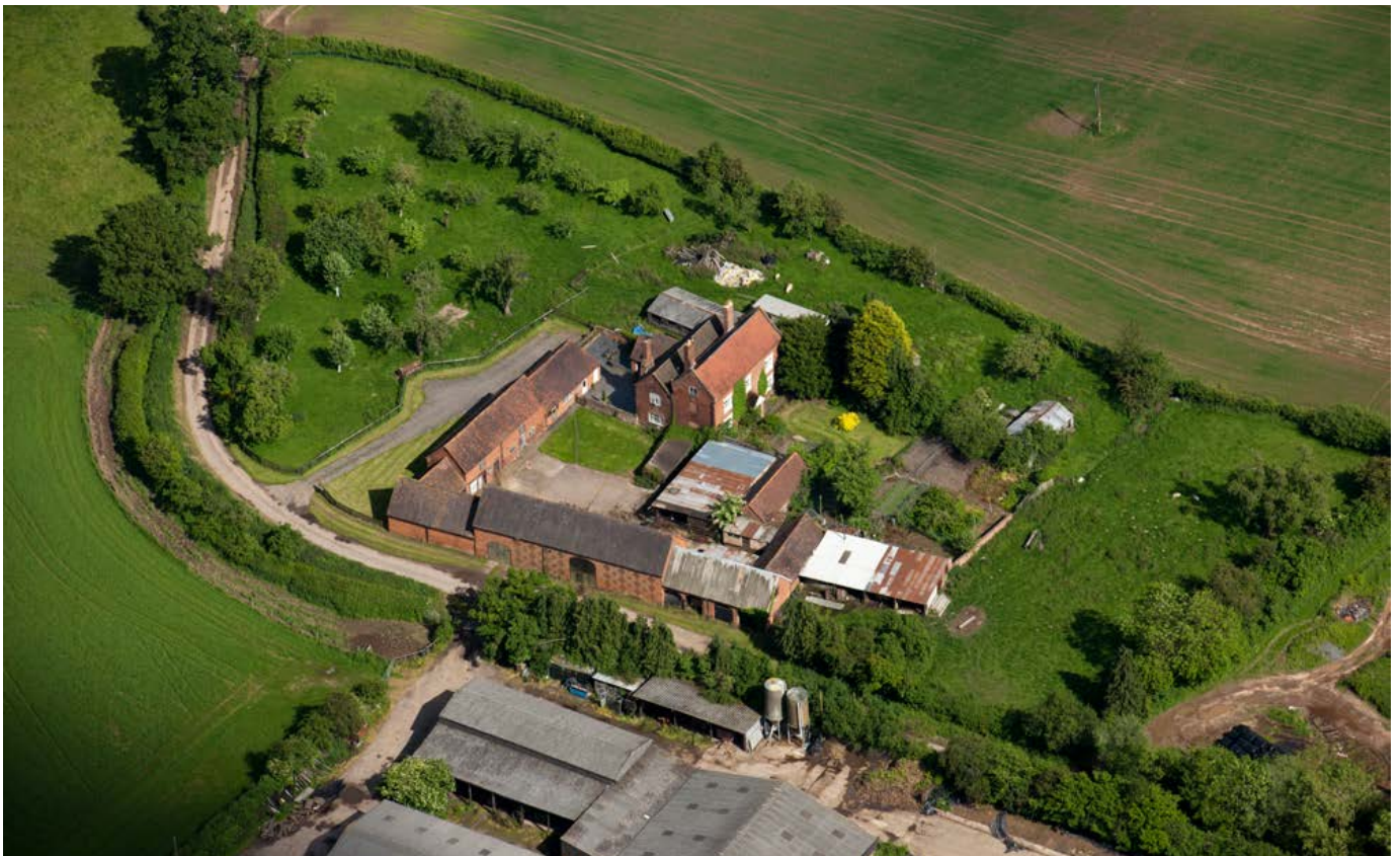
A regular courtyard farmstead near Enville with a late 18th-century farmhouse facing into its garden, with working buildings reflecting mixed dairying with arable production. To the rear of the house and its dairy are pigsties and calf houses. Attached to these are a two-storey cowhouse with a hay loft and a long hay and corn barn with stables facing the yard and a cart shed facing the road. Photo © Historic England 2900/03
