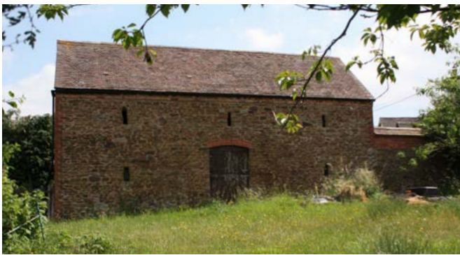
The rear of a small combination building with animal housing either side of a central passage which may have served as a threshing bay within the Wyre Forest. Photo © Bob Edwards
