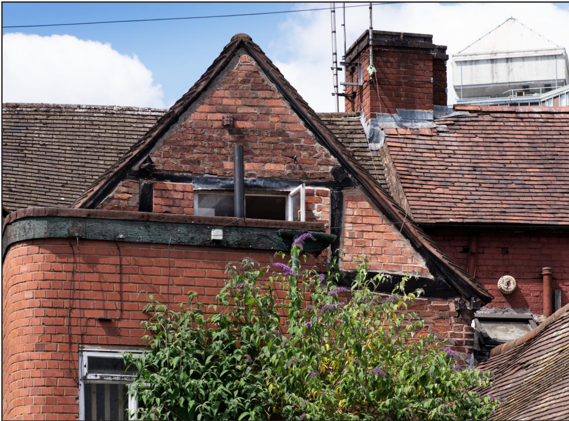
Figure 34: Timber framing to the rear of the Coventry Cross, as viewed from Palmer Lane, November 2019 (DP248430)
