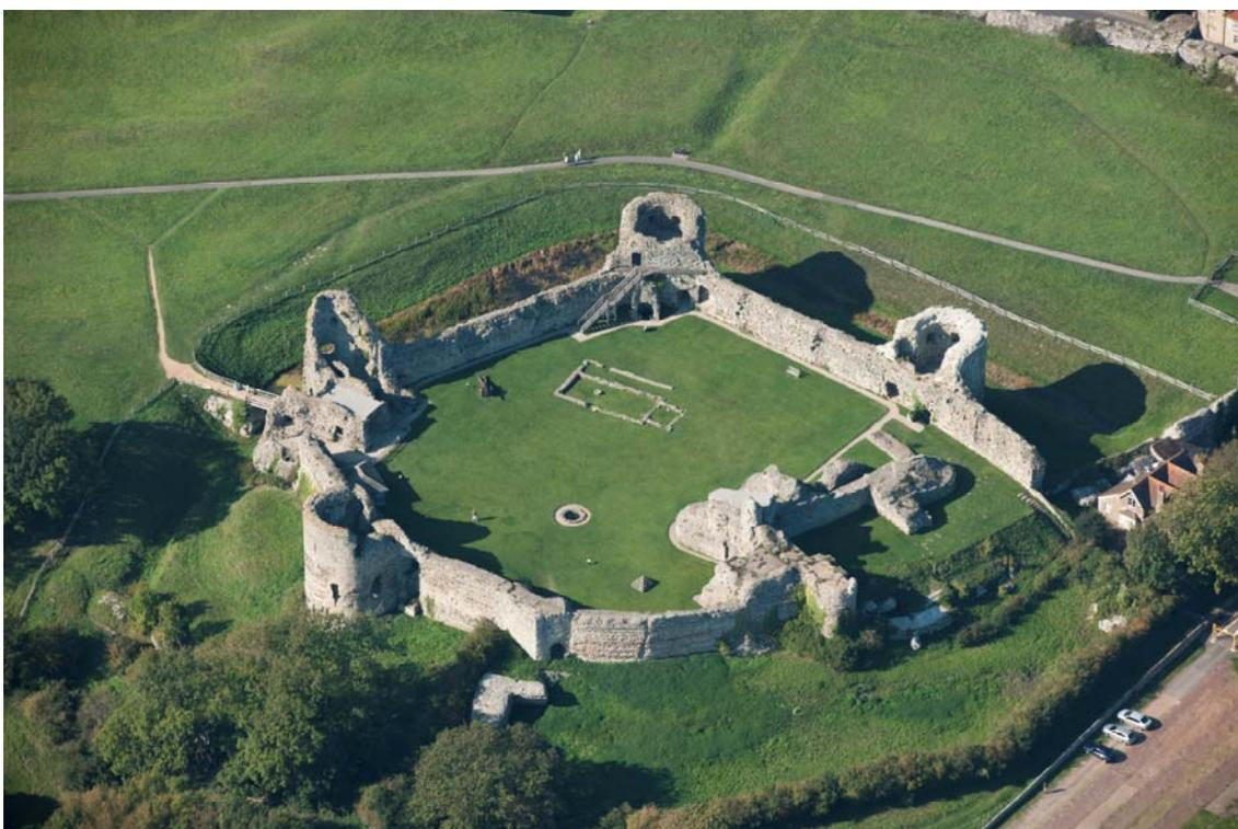
*Fig 12: The current chapel footings, in the centre of the image, probably date from the early 14th century, when documents refer to the construction of a new timber-framed chapel (NMR 27303/023 29-Sep-2011)*
