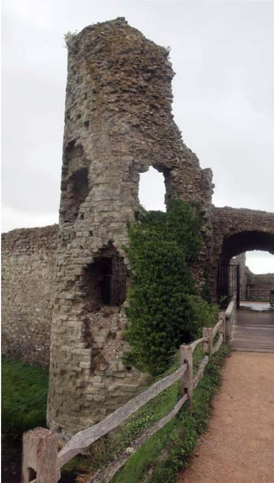
*Fig 17: The north turret of the gate survives to a large extent and illustrates that the stonework is of superior quality to the flanking walls of the castle (Investigator Photograph)*
