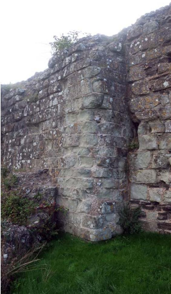
*Fig 7: Straight joint between the west side of the postern gate and the south wall of the medieval castle to the right (Investigator Photograph)*
