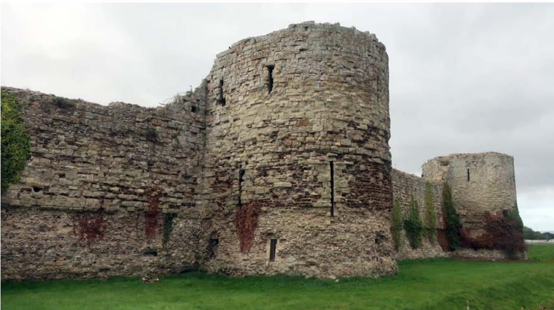
*Fig 16: Despite the robbing of the good quality ashlar of the lower courses on the north side of the castle, the walling seems a little neater and more sophisticated than the south side of the castle (Investigator Photograph)*
