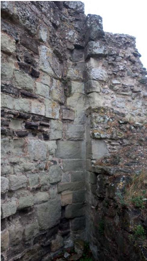
*Fig 13: There is a clear joint between the main gatehouse on the right and the rubble of the south wall of the medieval castle on the left (Investigator Photograph)*
