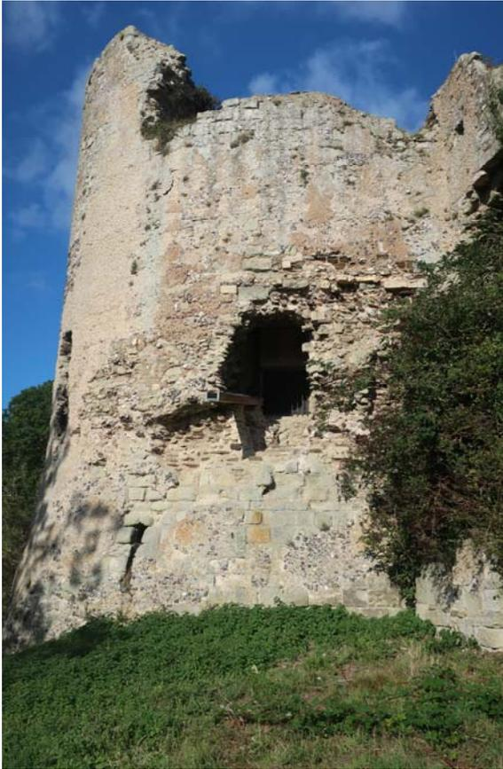
*Fig 15: Assessing the character of the walling on the south side of the medieval castle is complicated by undergrowth and more intrusive 20th-century interventions and repairs. Nevertheless, it seems to be somewhat coarser in finish than the west and north walls of the castle (Investigator Photograph)*
