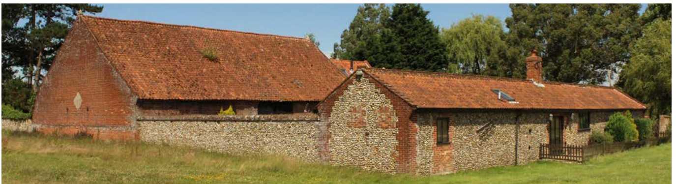
The late 18th-century brickwork to this five-bay barn at Brisely probably disguises an earlier timber-frame. It faces a cattle yard with brick dressing to flint walls. Photo © Bob Edwards
