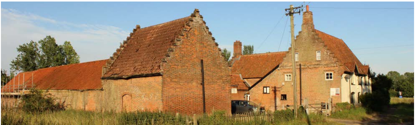
This 17th-century group at Morton on the Hill comprises one of the finest examples of Low Countries influence (the early use of brick and of crow-stepped gables) in the region. Photo © Steve Podd
