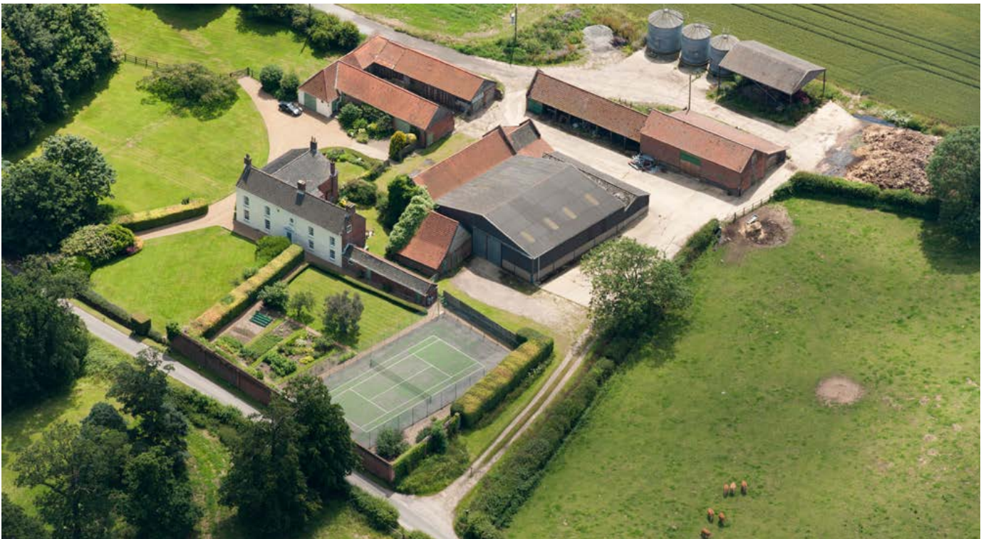
A regular multi-yard plan near Great Plumstead. The house and the threshing barn closest to it date from the mid- to late 18th century. All the other buildings including the other threshing barn were rebuilt in the early to mid-19th century, when the house was refronted to face its own garden facing away from the working yards. Photo © Historic England 29124/022
