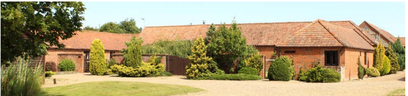
Extensive ranges of cattle buildings added to farmsteads, mostly of mid-19th-century date, as here, are another key characteristic. Photo © Bob Edwards
