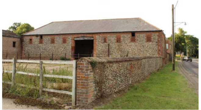
Decorative use of brick in ventilation slits and quoining is another feature, as at Dunton (left) and East Raynham (right). Photo © Bob Edwards
