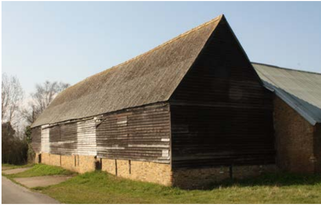
There are some larger barns within the Essex marshes. This barn of seven bays was originally timber-framed but has been largely re-built in brick in the 19th century. Photo © Bob Edwards
