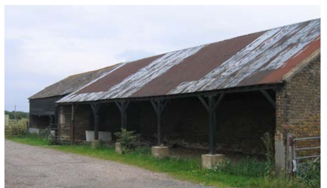
A cartshed forming part of a courtyard group with an L-plan range and a building to the third side of the yard. Typically, the cart shed faces out, away from the yard. Photo © Bob Edwards
