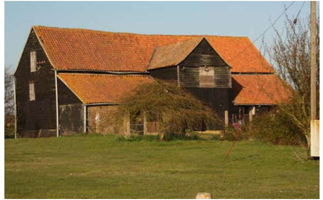
An early 17th-century five-bay barn on a high status farm in the Essex marshes. The later additions providing stabling or cattle housing. Photo © Bob Edwards
