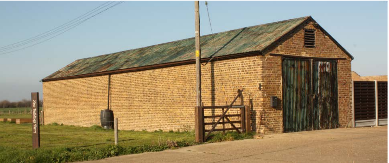
Sheds with gable end access are found on some farmsteads. These are usually of late 19th-century date. Photo © Bob Edwards
