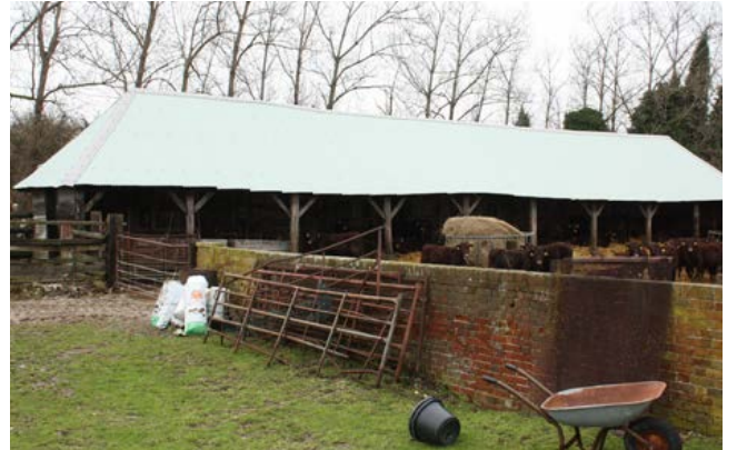
An open-fronted shelter shed, possibly of late 18th-century date. Most shelter sheds date from the 19th century. Earlier examples are rare. Photo © Bob Edwards
