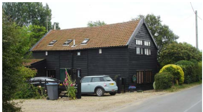
An 18th-century or earlier, three-bay threshing barn, typical of smaller farmsteads in its small scale and use of timber-frame in this area, now in residential use. Photo © Steve Podd
