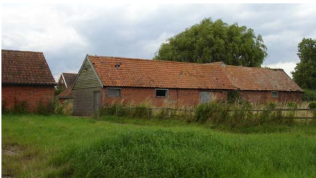
Mid- to late 19th-century housing including a sliding door as introduced onto farms from the 1850s. Photo © Steve Podd
