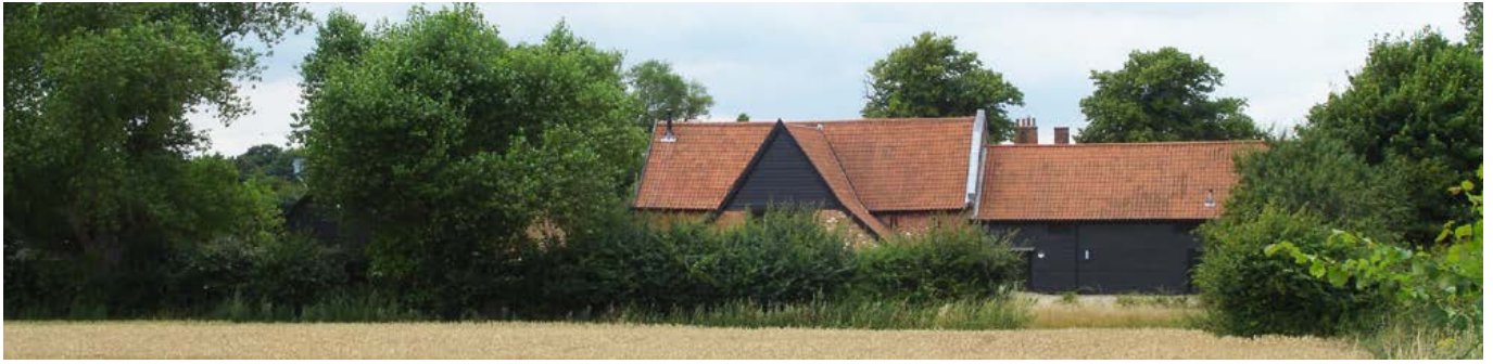
A late 18th-century threshing barn with a gabled porch, its brick construction typifying the rebuilding of farmsteads from the late 18th century in this area. Photo © Steve Podd
