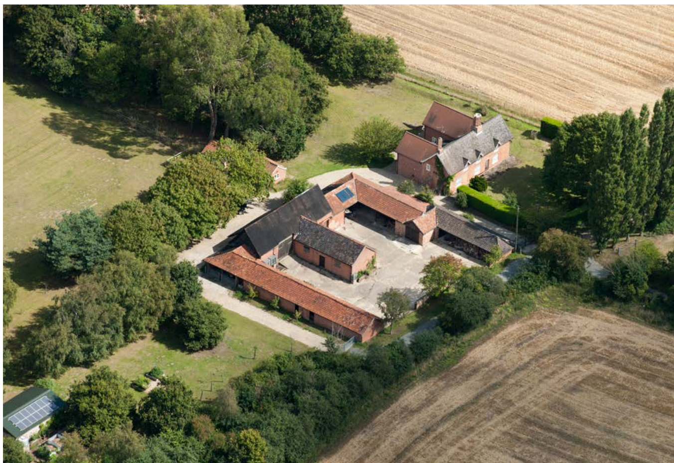
Early 19th-century barn with central threshing floor at Snape, with later lean-tos for housing cattle. Photo © Bob Edwards.
