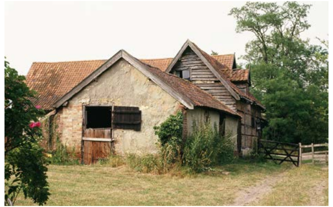
Rare example of 18th-century stables, built of timber-frame clad in weatherboard, attached to a small barn (to the left) and a cow house (to the right). The whole group is a rare example of pre-improvement farmstead architecture in this area. Photo © S Wade Martins
