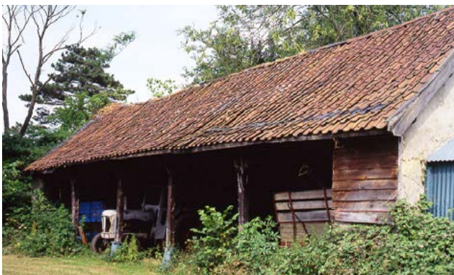
Cart shed, probably late 18th-century as built of light timber studding with clay walling. Photo © S Wade Martins
