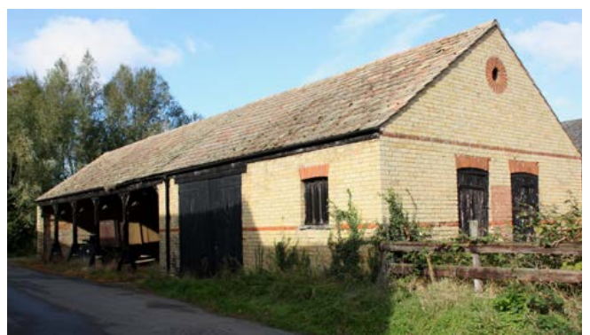
The use of yellow brick reflects the importance of the area's brickworks, as here combined with red brick detail in this stable and cartshed range in the south of the area. Photo © Bob Edwards
