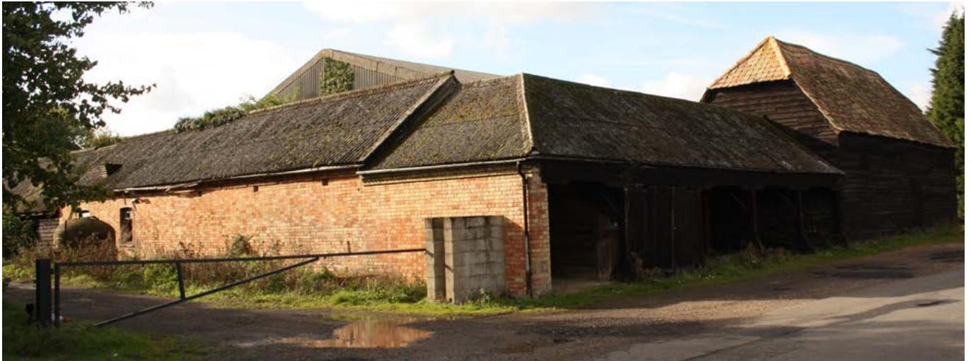
Early barns could also be integrated into large-scale regular courtyard layouts that mostly date from rebuilding in the early to mid-19th century. Here a relatively small-scale three-bay barn with a half-hipped roof (another distinctive characteristic of traditional architecture in the south-east of England and southern East Anglia) is attached to a large, five-bay cart shed that faces into the road and away from the internal cattle yard. Photo © Bob Edwards
