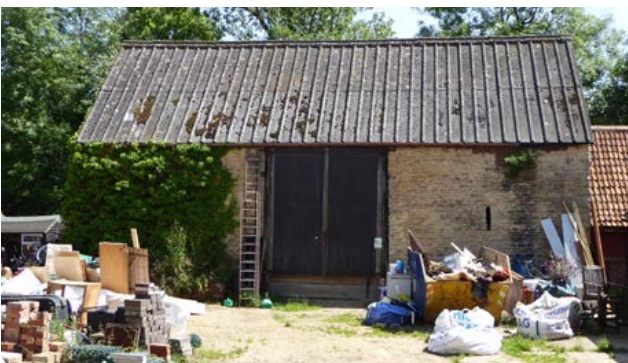
Three-bay threshing barns continued to be built, as here, on smaller farms into the mid-19th century. Photo © Jeremy Lake
