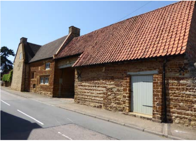
Whilst many farmhouses – long decoupled from agricultural use – remain within villages, surviving farm buildings are rare. These also can include, albeit surviving in a fragmentary state as here at Whiston, late 17th-century and even earlier fabric which indicates the growing property of farms which were subject to later programmes of rebuilding, as farms moved out of villages into enclosed fields. Photo © Jeremy Lake
