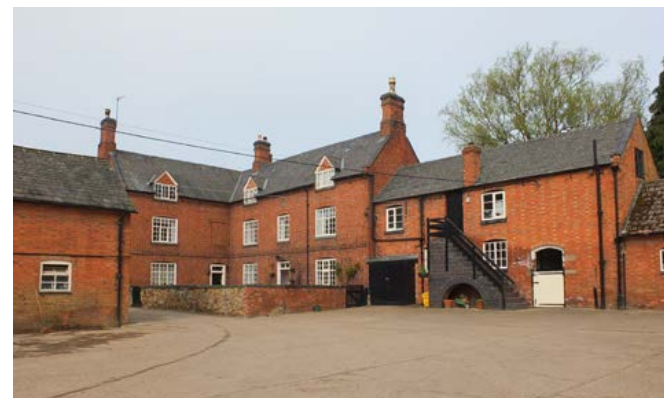
Cattle housing and dairy with louvred vents, and a farmhouse with an attached granary/stable range, forming part of a large, mid-19th-century farmstead. The farmstead is of a regular courtyard plan form as are many of this period and is built of brick. The design and the strong orange brick work of these outlying farms is a distinctive feature of the landscape and particularly noticeable in the west and towards the centre of the area. Photo © Jen Deadman
