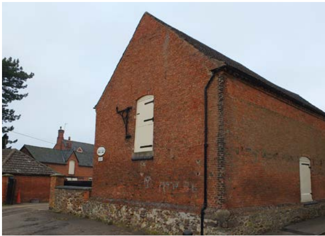
The early 19th-century combination barn at Manor Farm is built on a cobble plinth. Note the dentilled moulding at eaves level and the crane to the first-floor granary. Photo © Jen Deadman
