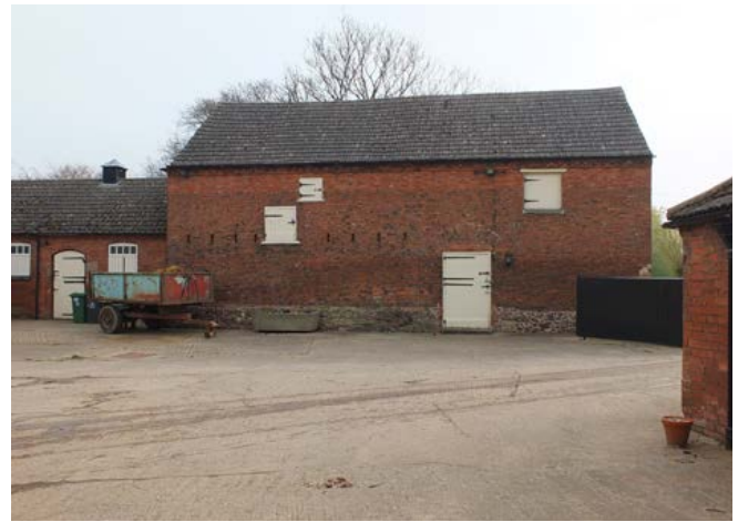
The early 19th-century combination barn at Manor Farm is built on a cobble plinth. Note the dentilled moulding at eaves level and the crane to the first-floor granary. Photo © Jen Deadman
