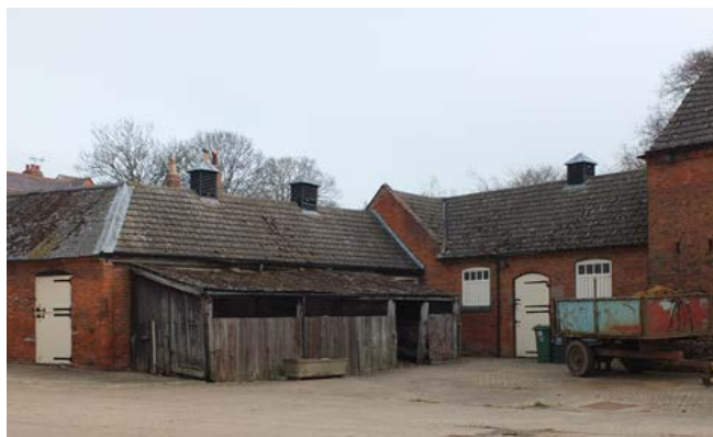
Cattle housing and dairy with louvred vents, and a farmhouse with an attached granary/stable range, forming part of a large, mid-19th-century farmstead. The farmstead is of a regular courtyard plan form as are many of this period and is built of brick. The design and the strong orange brick work of these outlying farms is a distinctive feature of the landscape and particularly noticeable in the west and towards the centre of the area. Photo © Jen Deadman
