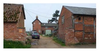
Surviving elements of timber frame and different phases of brick construction are visible in this farmyard facing the village street in Ashby Magna. Photo © Jen Deadman
