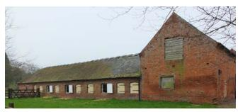
Raised ridge tiles and hatches for throwing out manure indicate a row of loose boxes, attached to a hay barn. Photo © Jen Deadman
