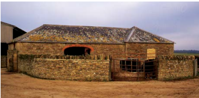
Many farmsteads were built with cattle sheds facing into yards with wide, arched openings, as seen here. These strongly resemble the hemmels seen in those areas of Northumberland where large-scale arable farming also developed. Photo © Jeremy Lake
