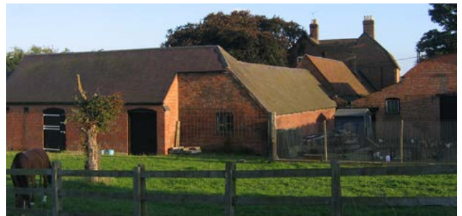
A regular plan farmstead where the buildings are interlinked, its low profile being typical of the Dunsmore area, where the rebuilding of farmsteads seems to have occurred at a later period in the 19th century than in Feldon. Threshing barns are rare, suggesting that this rebuilding occurred after the introduction of mechanisation. Photo © Jeremy Lake
