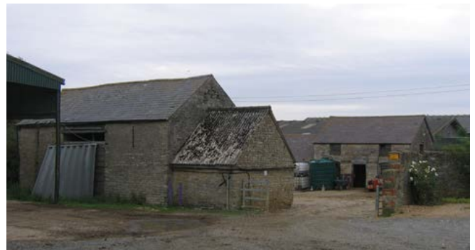
A loose courtyard plan built of Liassic limestone to the south of the Feldon. The early to mid- 19th-century threshing barn and (to the rear) the threshing barn testify to the importance of arable farming in this area. Photo © Jeremy Lake
