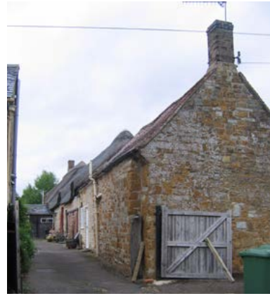
A linear plan farmstead in a village in the south of the area. Photo © Bob Edwards
