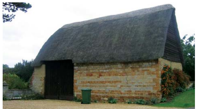
A rare surviving example of a small-scale threshing barn, refronted in the 19th century in a distinctive mix of banded lias and ironstone. Photo © Jeremy Lake
