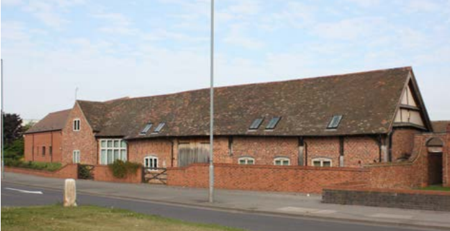
Barns were commonly extended and refronted in brick, as in this example, converted to residential use in the suburbs of Birmingham. The window openings are not purely domestic: it was common for barns to be converted into housing for dairy cattle in the late 19th century. Photo © Jeremy Lake
