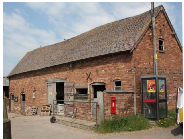
Large, multifunctional combination barns were commonly built in brick in the early to mid 19th century, and brought many functions together into a single building. This example includes a threshing barn flanked by a stable (right) and cattle housing at the lower end to the left. Photo © Jeremy Lake
