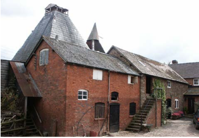
Many kilns for drying hops adjoin earlier, timber-framed structures, including some early kilns, which were converted into stowage rooms for storing and bagging up the dried hops. This brick building has an earlier timber-framed core. Photo © Jeremy Lake
