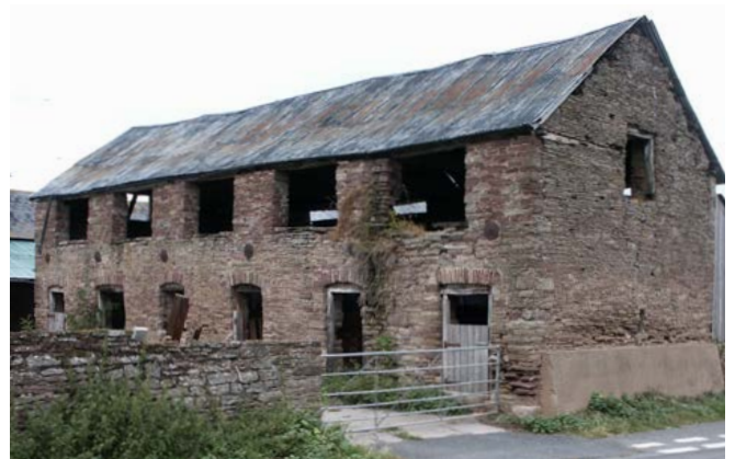
Some cow houses had open-fronted haylofts resembling the lincays of South Wales and South West England. Photo © Bob Edwards
