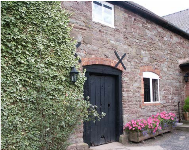
Cider houses are marked by wide doorways for moving barrels. Photo © Jeremy Lake
