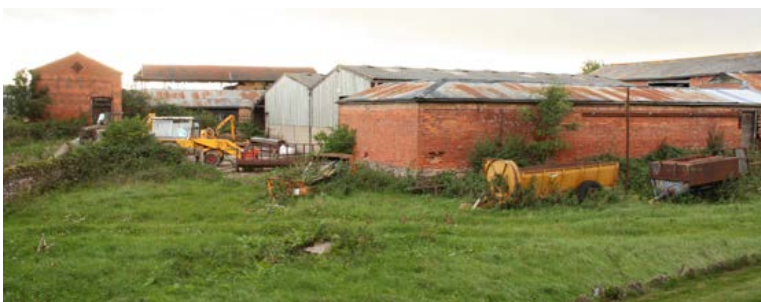
Preston Court is one of a number of large, isolated and high-status farmsteads sited on the terrace overlooking the flood plain of the Wye Valley, often positioned adjacent to the parish church. Photo © Bob Edwards
