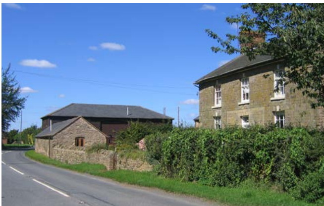
A symmetrically-planned three-bay house and L-plan farmstead of the early to mid- 19th century which occupies a roadside position within common land enclosed in the 19th century, on the eastern edge of the area. Farmsteads of this type are more commonly found in the Herefordshire Plateau to the north. Photo © Jeremy Lake
