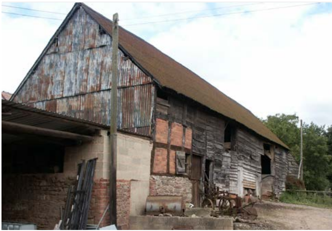
Large-scale, timber-framed barns had developed as a feature of this area by the 18th century, testifying to the large scale of farms that developed following widespread settlement change from the 14th century. This is a combination barn, with a cow house to one end of the threshing barn itself. Photo © Bob Edwards
