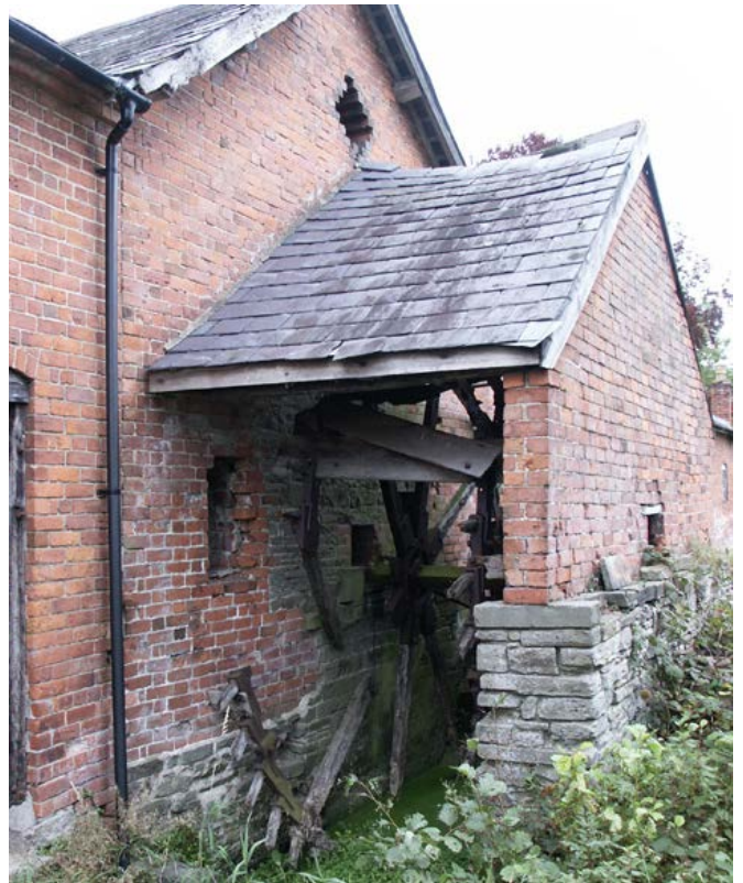
Water was used for flooding meadows and powering mills and barn machinery, as shown here. Photo © Bob Edwards
