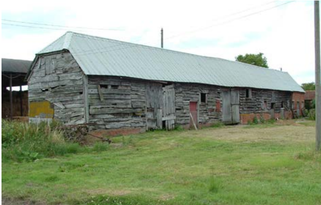
An example of a combination barn with storeyed cattle housing in timber-frame with weatherboard. The Teme Valley includes some very rare examples of 18th-century and earlier cattle housing, part of a distribution that is concentrated along the Welsh borders. Photo © Bob Edwards
