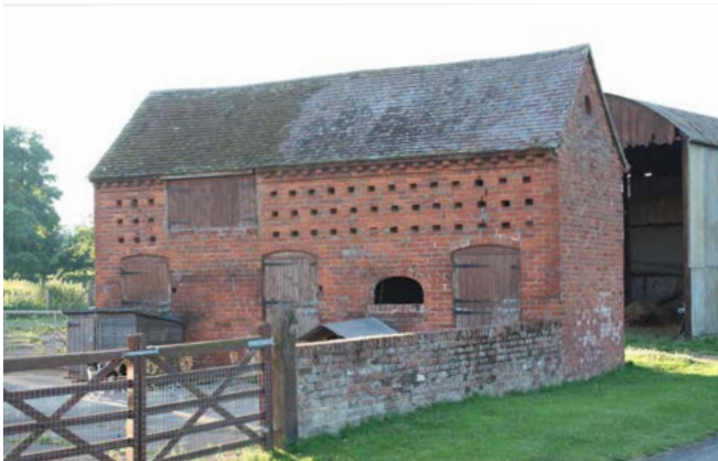
A cow house with ventilation holes marking the first-floor hay loft. Photo © Bob Edwards
