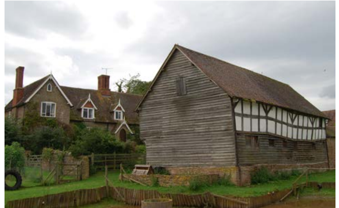
A two-storey, timber-framed cow house, this being a very rare survival. Photo © Worcestershire County Council
