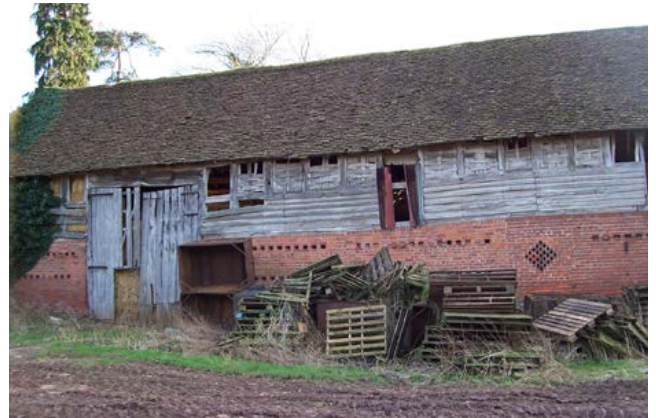
Timber-framed combination barns are common within this area. This barn (combined with cattle housing) has the characteristic woven panels to high level, a feature seen across Herefordshire with brick – possibly replacing framing – to the lower walls. Photo © Natural England
