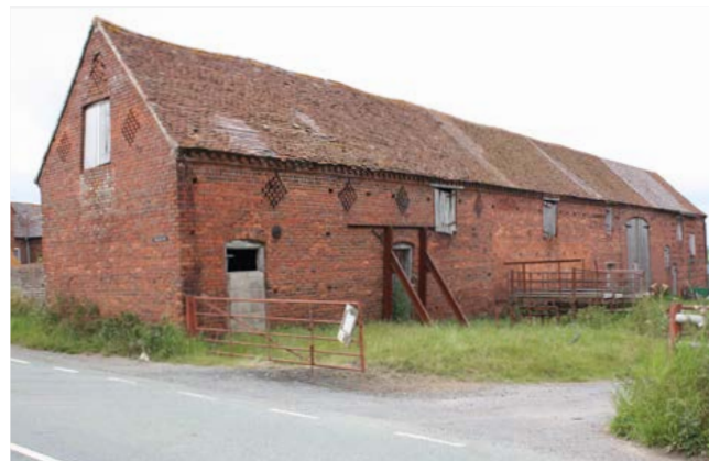
An early 19th-century combination barn with a cow house to the left and a threshing barn to the right. Photo © Bob Edwards
