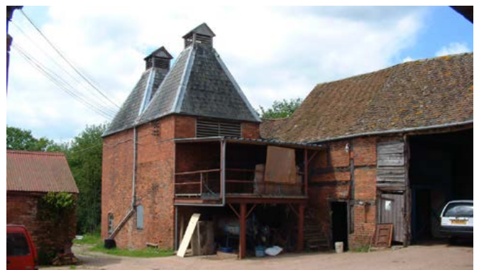
On many farmsteads, hop kilns were an addition to existing buildings in the late 19th century. Here, a timber-framed building serves as the stowage for dried hops adjacent to the kilns. Photo © Bob Edwards
