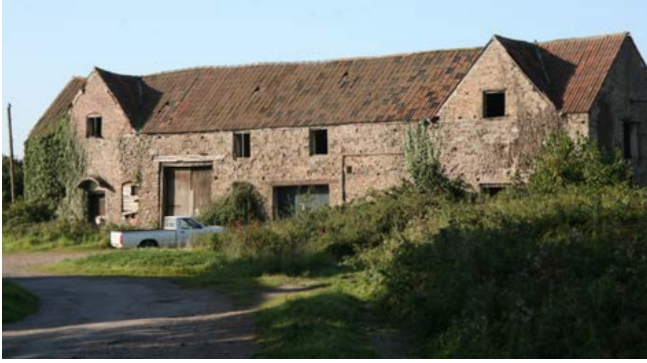
Another high-status example close to the River Severn, converted into cattle housing in the 19th century with the added brick gables. Photo © Sam Hale
