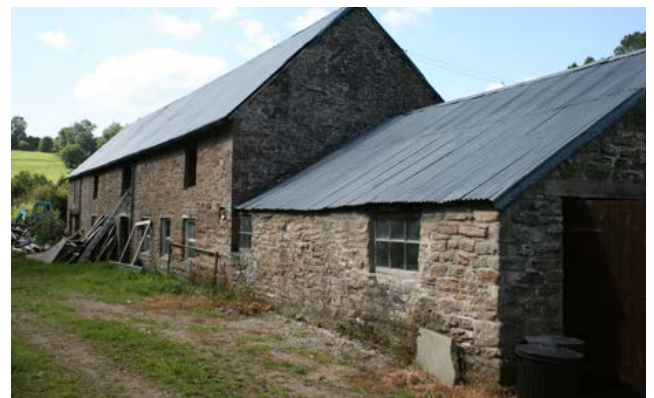
Cattle housing projecting from a multifunctional combination barn of early to mid- 19th-century date. Photo © Sam Hale
