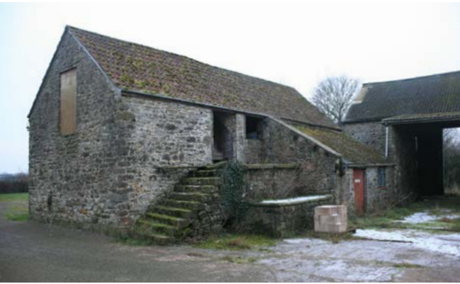
The corner of a farmyard with a first-floor granary marked by the steps, and a threshing barn to the right. Photo © Sam Hale
