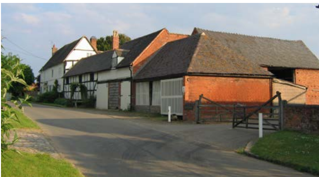
Large farmsteads often developed from the 14th century, close to the sites of farming settlements. This site near Worcester has a house, stable and large barn dating from the 17th century or earlier, reflecting changes still observable in the settlement change and piecemeal enclosure of the surrounding landscape. Photo © Jeremy Lake
