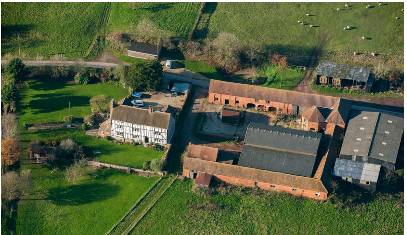
Large-scale farmsteads often developed around earlier houses, which testifies to the emergence of large farms between the 15th and 17th centuries, often intermixed with small-scale farmsteads. The regular courtyard U-plan here dates from the mid-19th century, the image showing a granary for storing grain and mixing feed above a cart shed range with stables to the left and a polygonal horse-engine house attached to the threshing barn to the right. Photo © Historic England 29237/041
