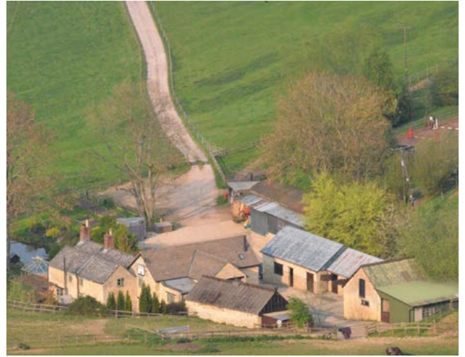
This farmstead has a loose courtyard arrangement with an early to mid-19th-century barn, stables, cattle housing and granary built around all four sides of the yard. Photo © Jeremy Lake
