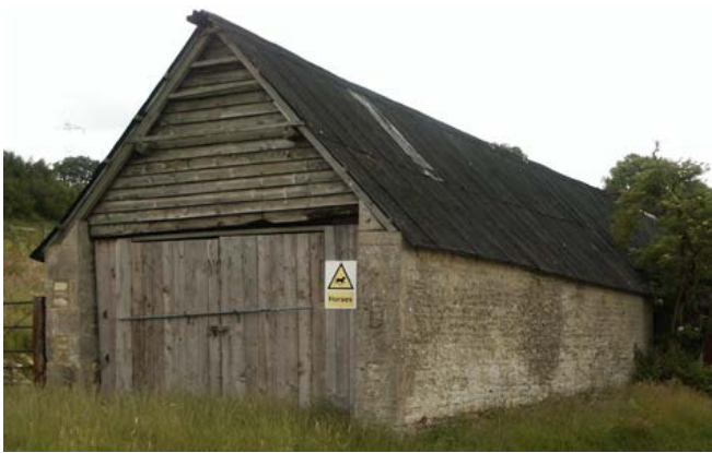
A cart shed. Cart sheds were often built with gable entries, as shown here. Photo © Jeremy Lake
