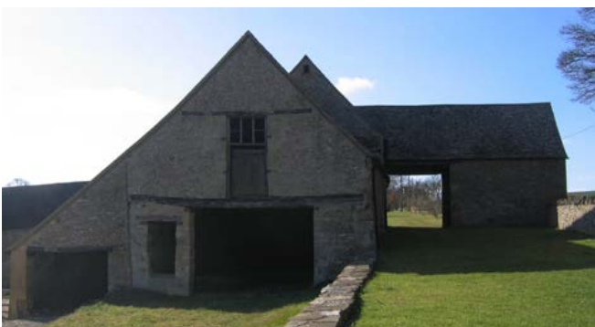
This large barn displays another commonly-encountered feature, which is the incorporation of a cart shed and stables into the barn and a throughway for offloading the harvested corn crop. Photo © Jeremy Lake
