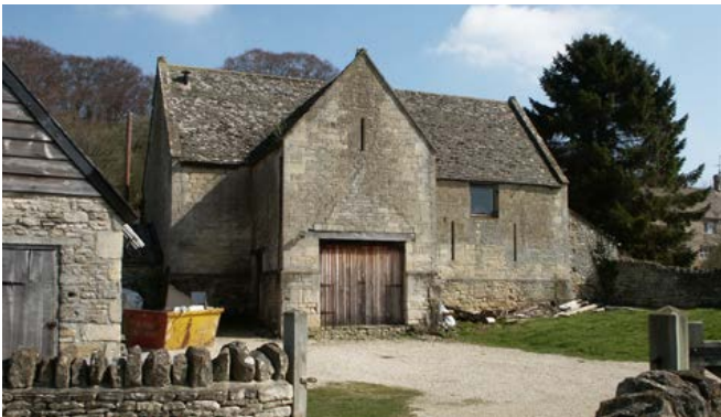
An early 19th-century barn, like many of this date, built with an off-centre threshing floor and also with the high-quality dressed stonework and stone-coped gables typical of Cotswold farmstead architecture. Photo © Jeremy Lake
