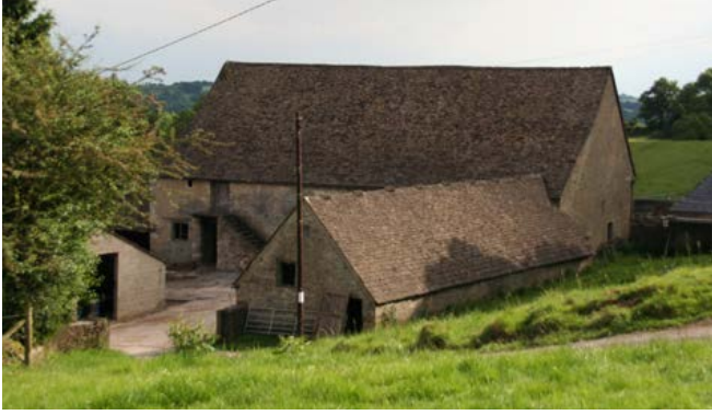
This L-shaped arrangement is typical of the Cotswolds, as also is the incorporation of the stable and its granary (with external stone steps) in the end bay of the threshing barn and the low cow house in the foreground. Photo © Jeremy Lake
