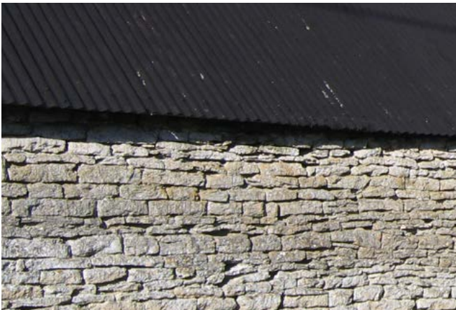
Many stone buildings display evidence for phasing in their construction. Corrugated iron was used in this area from the late 19th century. Photo © Jeremy Lake
