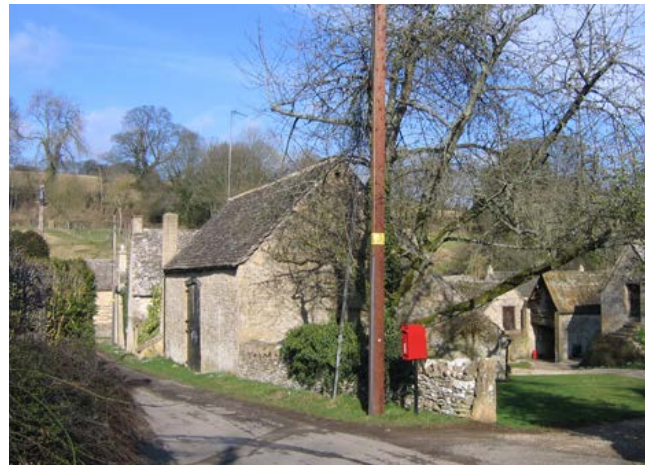
View into a village farmstead at Duntisbourne Abbots north of Cirencester. Buildings from the 17th to 19th centuries include a threshing barn facing the road and a granary served by steps. Photo © Jeremy Lake
