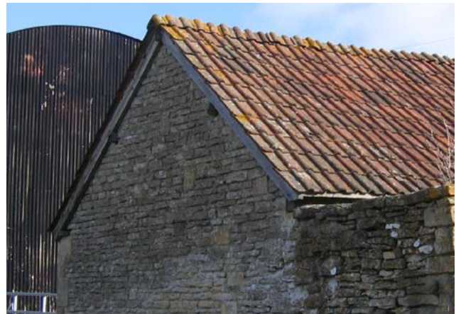
Roman tiles and plain tiles were used, but in limited numbers. Photo © Jeremy Lake
