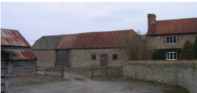
A combination barn which incorporates a threshing barn and stable along the southern fringe of the Midvale Ridge, again with its characteristic combination of stone rubble walling and clay tile roof. Photo © Jeremy Lake
