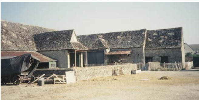
The L-shaped range of barns at Cogges Manor, Witney, developed over the late 17th and 18th centuries, leaving the much smaller 17th-century barn (right) to be converted into a stable. This type of development is repeated across the area. The building materials are typical for the limestone belt. Photos © Jeremy Lake
