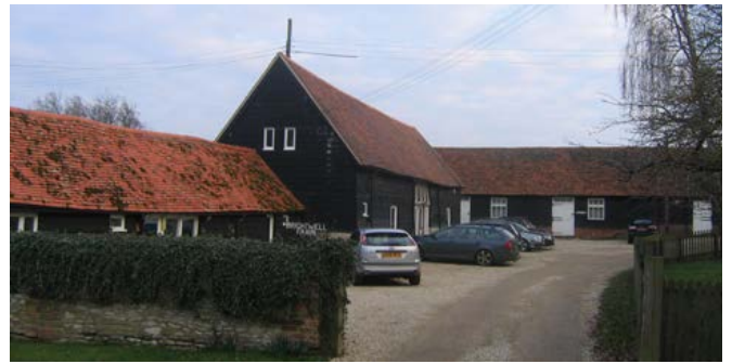
Many courtyard farmsteads developed around three or four sides of the yard. This example in the south of the area, in weatherboarded timber frame and tile, has two sides of the yard covered by an L-plan range with a barn and flanking stables and cattle housing. Photo © Jeremy Lake
