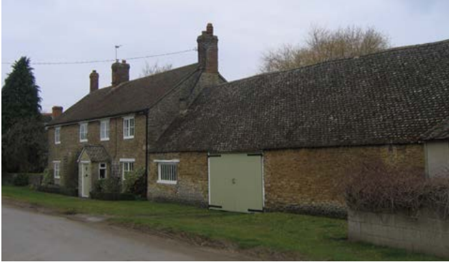
Working buildings within settlements were frequently attached to farmhouses, a feature of farmstead planning found elsewhere in the villages of the limestone belt. The house typically faces the main routeway, and to the rear is the main yard. Photo © Jeremy Lake
