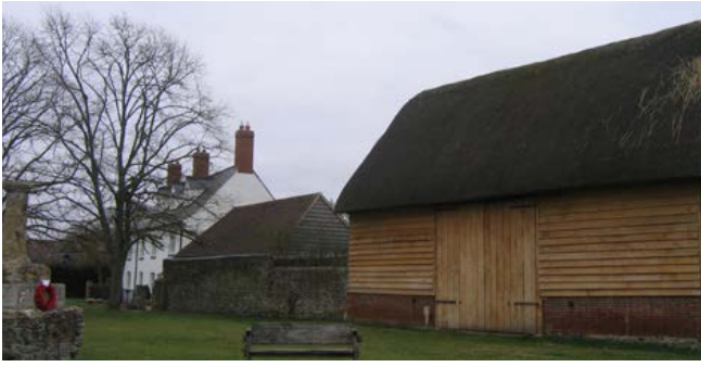
A timber-framed barn with a thatched roof in Charney Bassett to the south of the Midvale Ridge, where the use and survival of timber frame increases. Photo © Jeremy Lake
