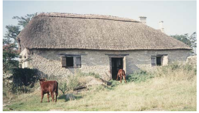
This oxhouse is an extremely rare example of a building for draught oxen, which had been replaced by horses over most of this area by the 18th century. Photo © Jeremy Lake
