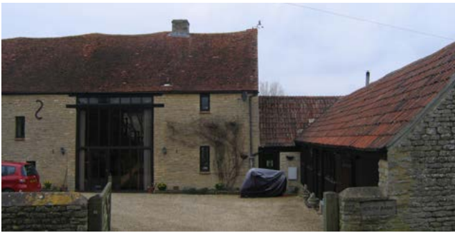
This example in the hamlet of Cote has shelter sheds for cattle attached to the threshing barn, again forming an L-plan in the corner of the yard. Note the use of clay tile with limestone rubble walls, a typical feature on the southern fringe of the Midvale Ridge. Photo © Jeremy Lake
