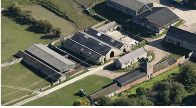
This farmstead was provided with a covered yard in 1858, soon after this innovative farmstead plan – which housed fatstock cattle and conserved their manure from the elements – was introduced during the so-called ‘High Farming’ period of the mid 19th century. Photo © Historic England 27293/028
