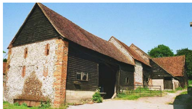
Piecemeal development of barns, as in other downland areas reflecting the need to house more corn as farms expanded in size, is another distinctive feature. At the far end is a barn built in timber frame with brick infill, with an outshot clad with weatherboarding for housing farm animals (probably a bull). The late 18th- and early 19th-century barns in the foreground used another commonly found combination of flint with brick dressings and timber-frame with weatherboard for the side walls. The clay tile roofs are another highly distinctive feature of the Chilterns. Photo © Chilterns Conservation Board
