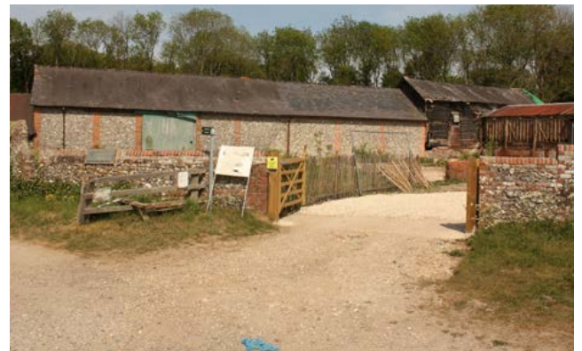
Most stables are 19th century and were built in flint and/or brick, sometimes with lofts for hay and storing grain. Photo © Bob Edwards
