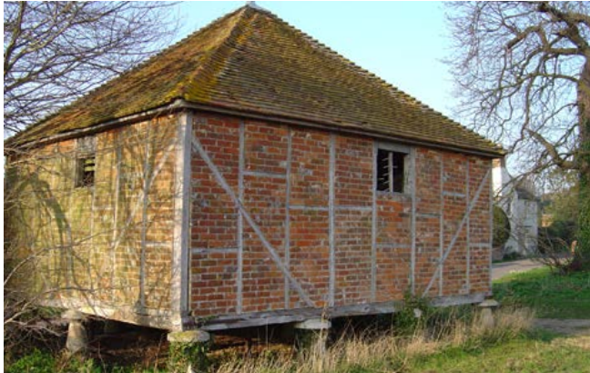
A granary on staddle stones. These were built in great numbers in the later 18th and early to mid-19th centuries, but have been vulnerable to change. Photo © Chilterns Conservation Board
