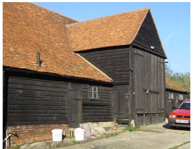
A typical threshing barn, with side aisles flanking the porch. Note the gap below the porch doors, into which would have fitted removable boards for use during threshing. Photo © Chilterns Conservation Board
