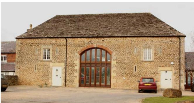
An early 19th-century threshing barn built in ironstone with stone-slate hipped roof on a larger farmstead. Internally, the walls of the barn are lined in brick. The farmhouse, attached to the left, is of c.1840. This barn was a multifunctional building; the smaller doors are original features. Photo © Bob Edwards
