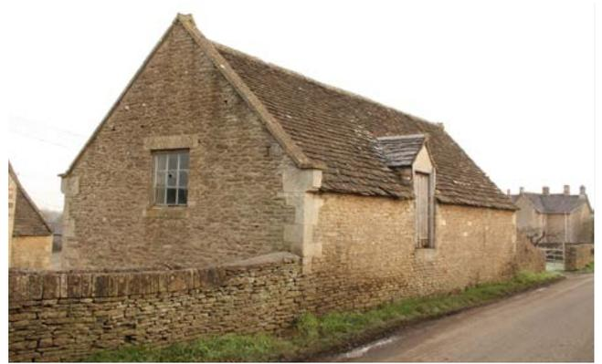
Large stables are not common in this area due to the limited extent of arable; only the larger farms having substantial stables. This example is of two storeys with the hay loft accessed from the road, which is higher than the yard, and a cart shed accessed from the far gable end. Photo © Bob Edwards
