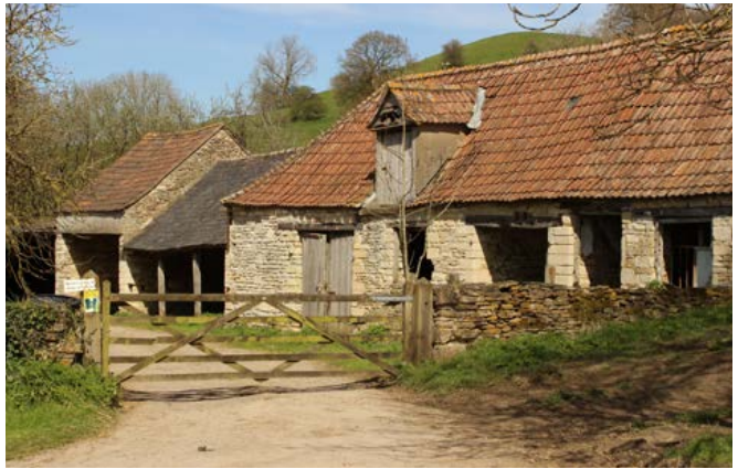
A small farmstead with its buildings set in a long row. These include an unusually small barn flanked by a shelter shed for cattle attached to a hay barn (to the left) and a granary over stables to the right. Photo © Bob Edwards
