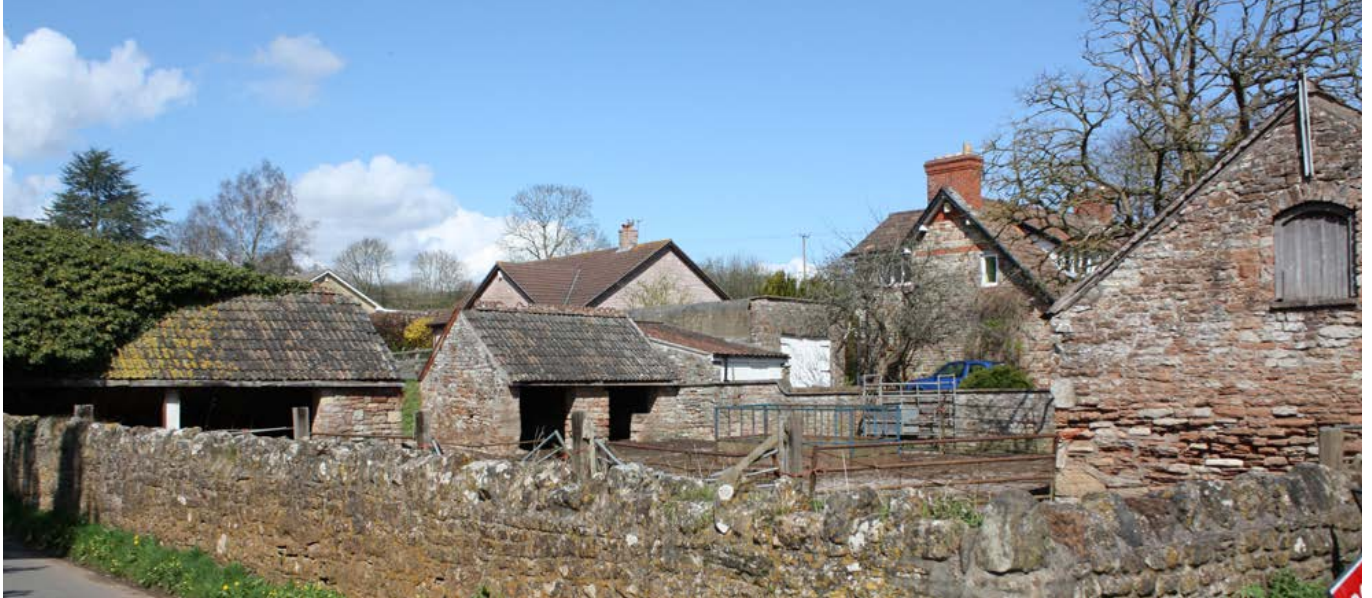
A small, mid-19th-century loose courtyard group with two small shelter sheds for cattle and a lofted cow house. Photo © Bob Edwards
