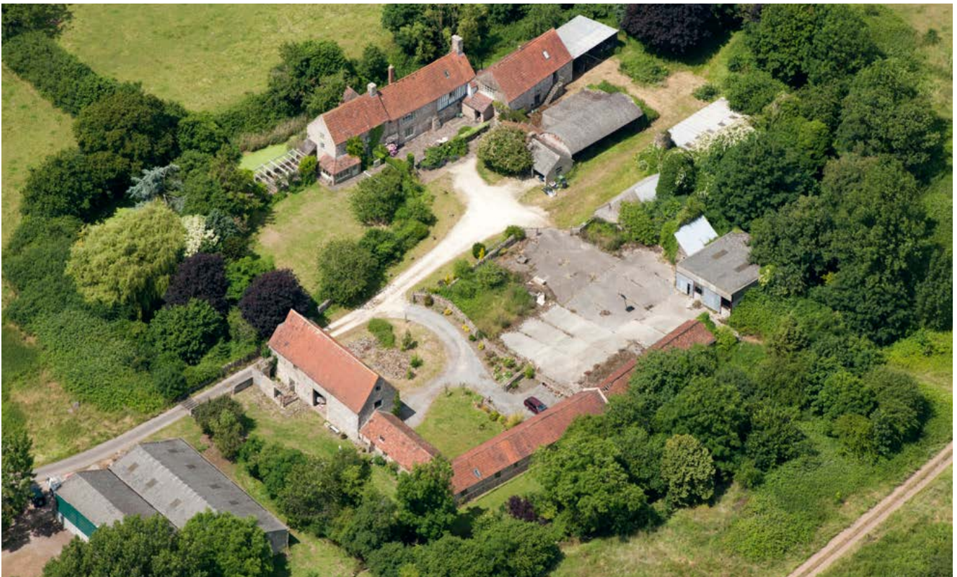
Yate Court is a medium-scale courtyard-plan farmstead with a five-bay barn, stabling and a long range of cattle shelter sheds, reflecting the importance of cattle on many farms in this area. The site dates from at least the 13th century. The medieval house stands close to an 18th-century or possibly earlier stable with steps to an upper-floor granary and detached bakehouse/brewhouse. The 16th-century barn to the bottom left is attached to an L-plan, 19th-century cattle yard. Photo © Historic England 29096/045
