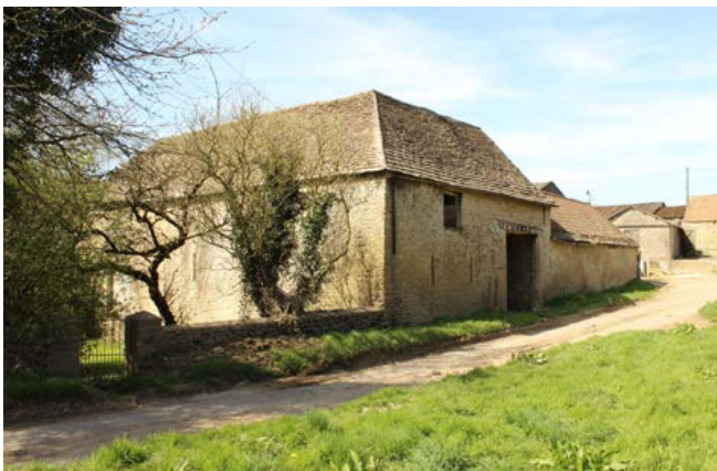
This large farmstead has a covered entrance into the yard with the 18th-century or earlier threshing barn set at right angles to the road. The end bay of the barn at least has a hayloft at upper floor level. Single-storey cattle housing backs onto the road. Photo © Bob Edwards
