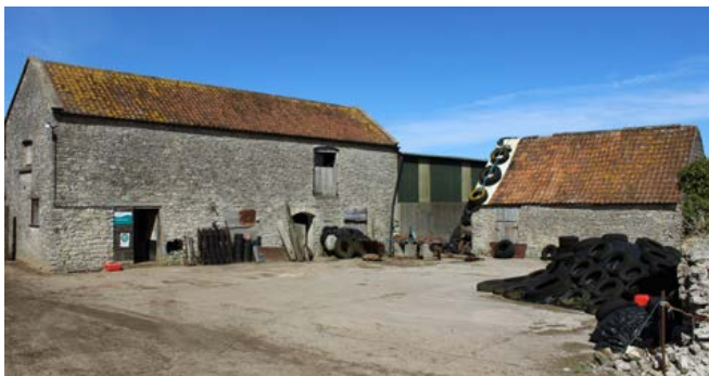
A loose courtyard group with late 18th- or early 19th-century buildings to two sides of the yard – a lofted cow house and a smaller building which may provide some stabling and storage. Photo © Bob Edwards
