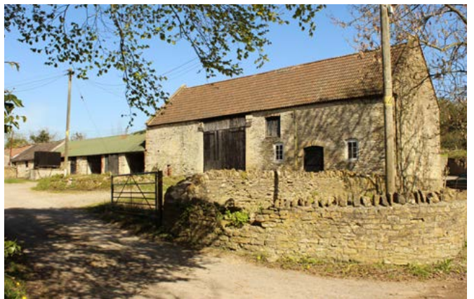
This combination barn range has a threshing barn of probably three bays with a lofted stable to the right. Photo © Bob Edwards
