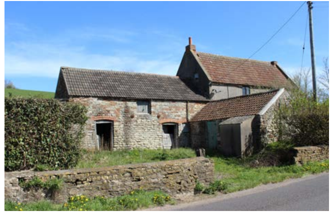
A small number of linear plans can be found in this area, typically with cattle housing attached to the farmhouse. This example is of late 18th- or early 19th-century date. Photo © Bob Edwards
