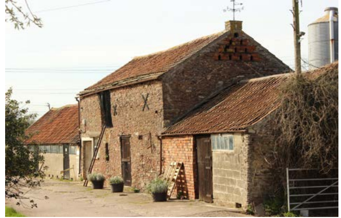
A two-storey stable with a hayloft over the stables. Nest boxes for pigeons have been built into the upper part of the gable. Photo © Bob Edwards
