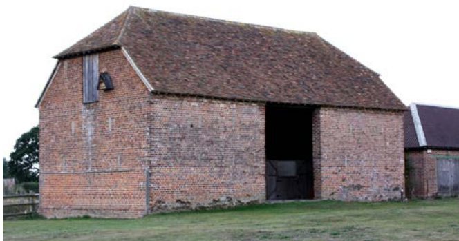
Brick-built barns are relatively uncommon in the North Downs. This example is probably of late 18th or early 19th-century date. Photo © Bob Edwards
