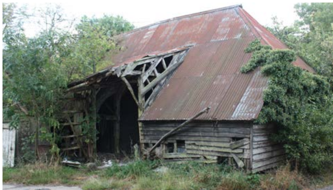
A three-bay barn, aisled to the front, with a hipped roof. Small-scale examples such as this are rare. Photo © Bob Edwards
