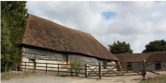
A large threshing barn on a high-status farmstead. The threshing bay has been blocked. Photo © Bob Edwards
