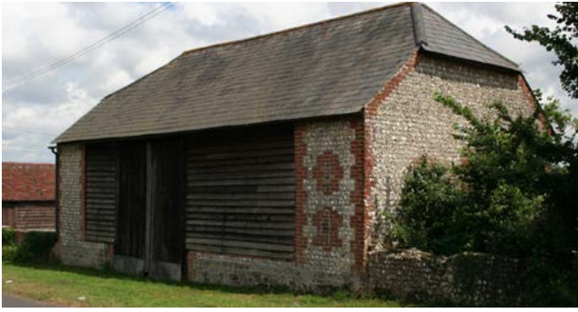
In areas close to the chalk of the Downs, flint was available which was combined with brick. This 19th-century barn also used timber-framing. Photo © Bob Edwards
