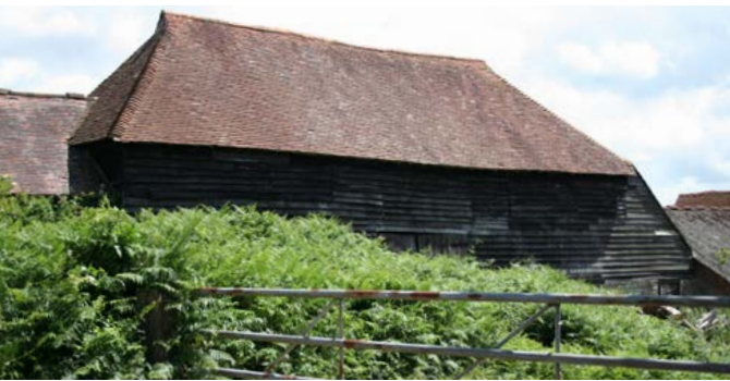
There is a good survival of timber-framed threshing barns in the Character Area, typically of five bays and with hipped or half-hipped roofs. Photo © Bob Edwards
