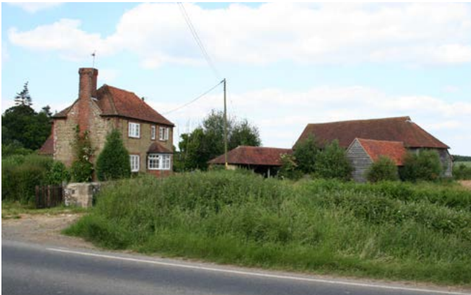
The small, U-plan range of this farmstead has a shelter shed and a stable attached to the barn and may be the result of later additions to an earlier barn. Photo © Bob Edwards
