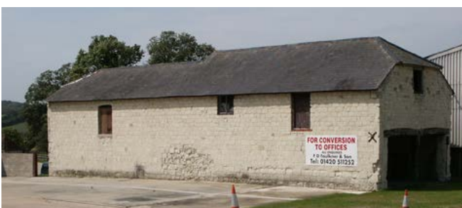
A cart shed and granary in the western part of the Character Area, where the sandstone, locally known as malmstone, is almost white in colour. Photo © Bob Edwards
