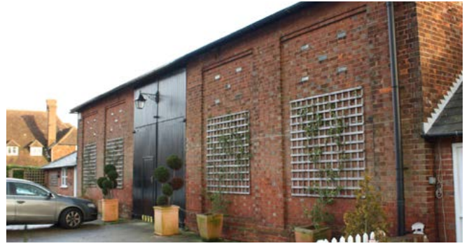
Brick was not widely used on its own for barns, usually being combined with stone. This five-bay barn was constructed in the early 19th century as part of a U-plan farmstead. Photo © Bob Edwards
