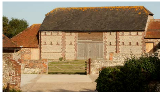
A five-bay, 19th-century barn built of cobble with brick dressings and having a half-hipped slate roof. Photo © Bob Edwards
