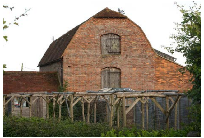
An unusual mansard type roof on this possibly three-storey 19th-century building. Photo © Bob Edwards
