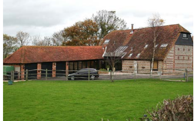
A regular L-plan consisting of a threshing barn with an attached, single-storey range which was probably a shelter shed for cattle. Photo © Bob Edwards
