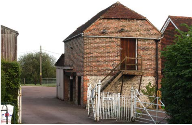
A small stable with a granary above. Photo © Bob Edwards
