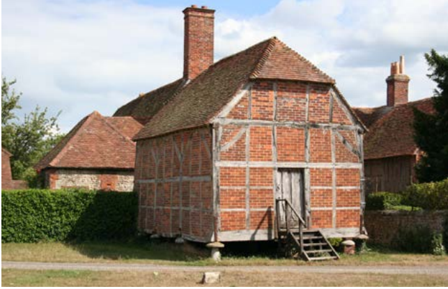
An early example of a timber-framed staddle granary, possibly of 17th-century date, with brick infill panels, located on a large manor farm. Photo © Bob Edwards
