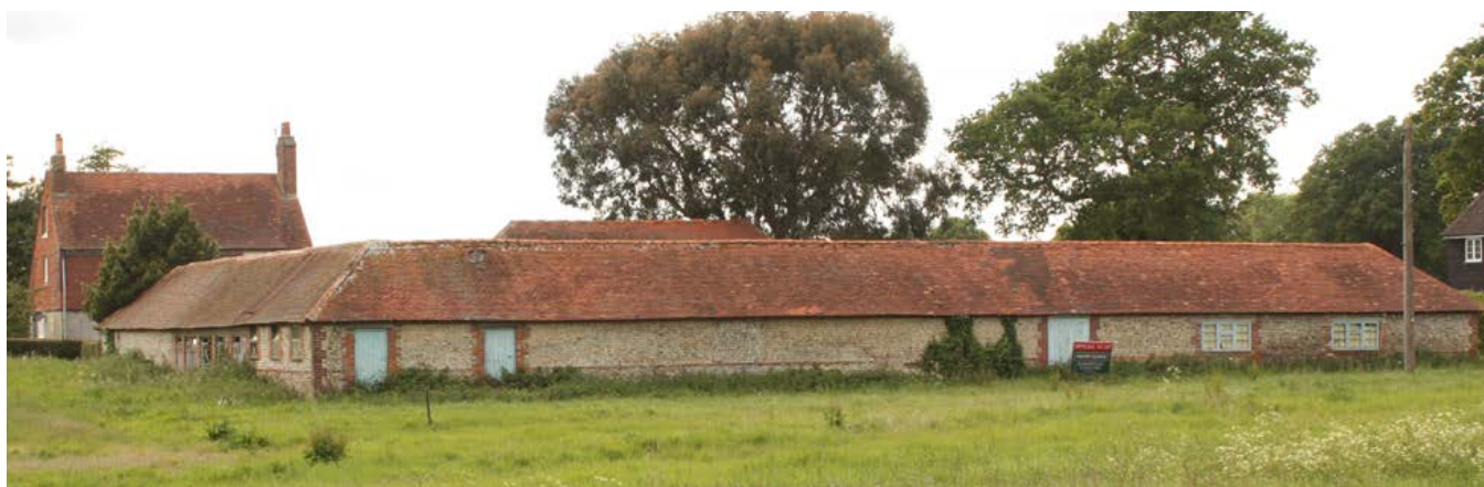
A courtyard plan with an L-plan range providing shelter sheds for cattle and stabling with a barn (its roof just visible) to the third side of the yard. Unusually, the house is attached to the L-plan range. Photo © Bob Edwards
