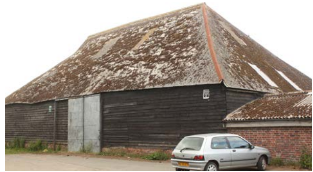
Five-bay barns are typical across the area, as in this aisled barn. Photo © Bob Edwards
