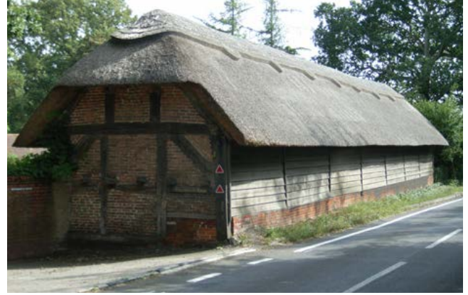
This 16th-century timber-framed building probably comprises a threshing barn with attached stable, a rare surviving example of its type. Photo © Bob Edwards
