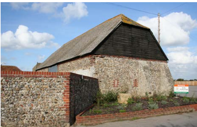
Cobbles from the beach were widely used for farm buildings, particularly in the 18th and 19th centuries. This five-bay barn retains timber-stud work above eaves level and has a half-hipped roof rather than the hips of earlier barns. Photo © Bob Edwards
