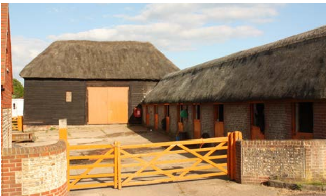
A small, three-bay, timber-framed threshing barn with an attached stable range. Photo © Bob Edwards
