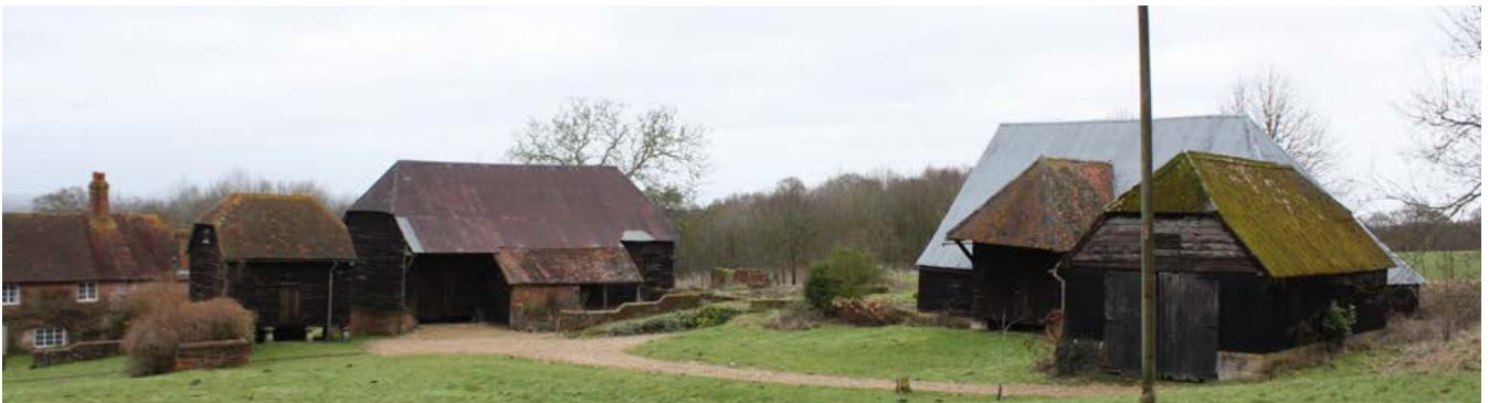
Loose courtyard plans with detached buildings set around a yard were the predominant farmstead type across the Character Area. Photo © Bob Edwards
