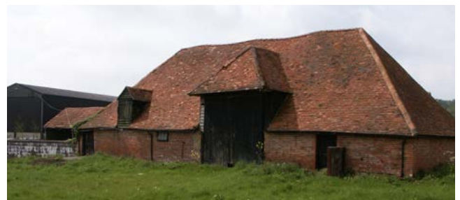
Barns in this wood pasture landscape are typically of three to five bays. This 17th-century, aisled barn has rebuilt aisle walls. The hayloft door at the far end indicates that this was a multifunctional barn with a floored bay and probably animal housing. The hipped roof is an important element in the character of this building. Photo © Bob Edwards
