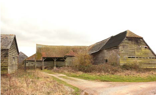
Within the river valleys, larger farms are to be found. This farmstead has an L-plan range of barns. The barn in the foreground is a 17th or early 18th-century, five-bay barn, aisled to the rear. The far range consists of a 16th-century, three-bay building that was originally floored throughout and was converted to a barn with the addition of bays at either end and aisles to both sides, probably in the early 19th century. Photo © Bob Edwards
