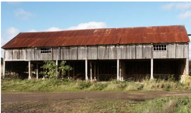
A late 19th- or early 20th-century cart shed and granary, its size indicating the importance of arable cropping in this area. A hatch over one of the bays allowed sacks of grain to be lowered into a waiting cart. The roof was almost certainly originally constructed for corrugated metal sheet. Photo © Bob Edwards
