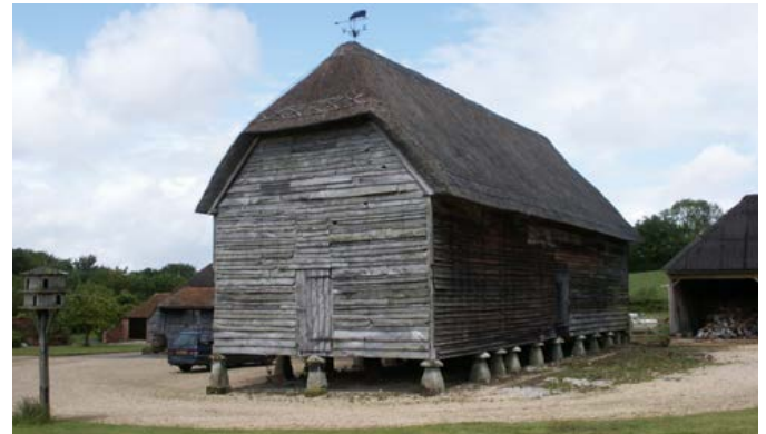
A staddle barn, a type of threshing barn that appears to have only been built in the decades around 1800 and is concentrated in west Berkshire and west Hampshire. Photo © Bob Edwards
