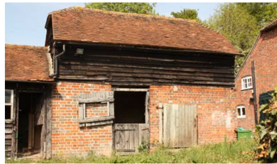
A small, early 19th-century stable with a hay-loft over on a small farmstead. Photo © Bob Edwards
