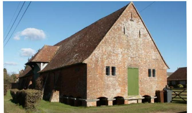
An unusual example of a granary built into the end of a barn, the brick arches providing ventilation below the granary floor. Photo © Bob Edwards
