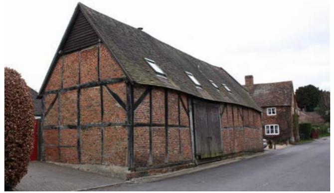
A 17th-century, three-bay, timber-framed barn with a central threshing floor (marked by the large double doors) has later brick infill and an added bay to the far end. Photo © Bob Edwards
