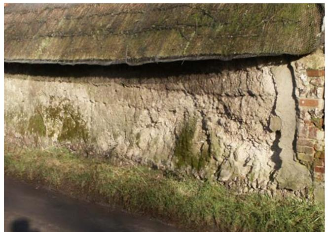
Cob boundary walls to farmsteads are an important feature in many of the valley-based villages. The cob was built off a flint or brick plinth and needed to be capped, either thatch or clay tile, to prevent water getting into the wall and often the cob was left exposed or covered with a chalk slurry. Photo © Bob Edwards
