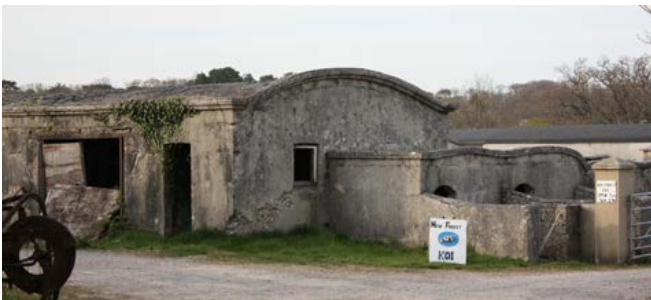
Piggeries built in mass concrete with vaulted roofs built c.1880 for A.T.T. Peterson who made important experiments in the use of this material. Photo © Bob Edwards
