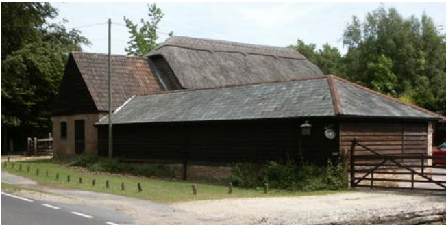
A regular L-plan created by the linking of a 19th-century shelter shed and an earlier timber-framed barn. Photo © Bob Edwards
