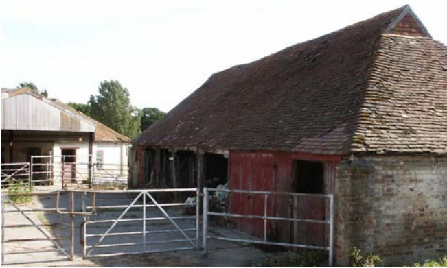
Shelter shed with plain clay tile roof. Photo © Bob Edwards
