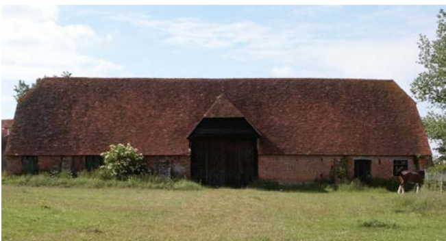
A five-bay threshing barn, probably of 17th-century date within the agriculturally fertile southern part of the Character Area. The Beaulieu estate added further ranges to enclose the yard beyond the barn in the late 19th century. Photo © Bob Edwards
