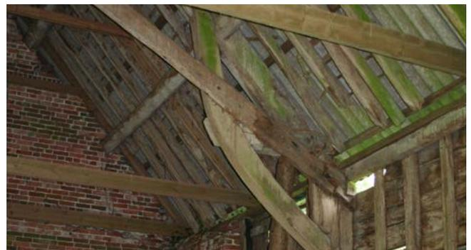
A barn with a 'sling brace truss': a 19th-century truss type that is rarely seen outside of Dorset. The diagonal timber is a later addition. Photo © Bob Edwards
