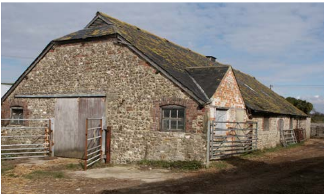
A late 19th-century, wide-span cattle shed effectively providing a covered yard where the cattle were sheltered from the weather and their manure protected from dilution by rain. The louvred ridge vent and vents at the gable provided ventilation. Photo © Bob Edwards
