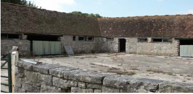
A cattle yard on a large farm defined by single-storey, 19th-century buildings which were partly open-fronted and which had been largely blocked with later infilling. Photo © Bob Edwards
