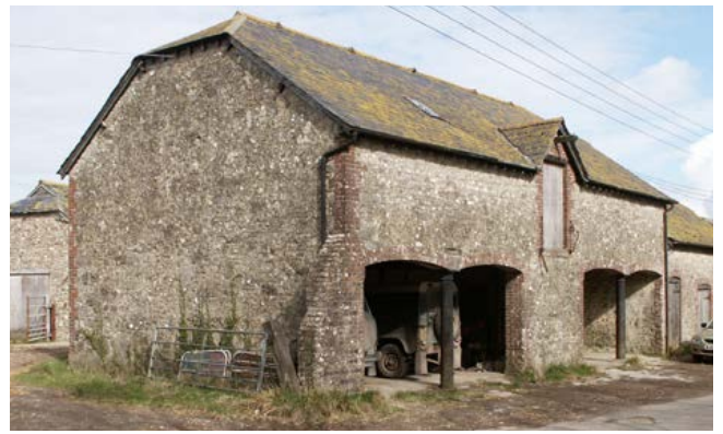
A late 19th-century cart shed with a granary above – the arm of a winch for raising and lowering sacks of grain survives above the loft door. The cart shed bays are divided by cast-iron columns. A small stable building is attached to the gable of the cart shed. Photo © Bob Edwards
