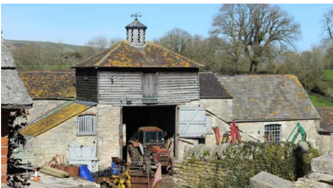
A dovecote incorporated into is what effectively the porch of a threshing barn with two lean-to buildings, probably for stabling or cattle either side, creating a relatively formal, designed appearance to this mid-19th-century building. Photo © Bob Edwards
