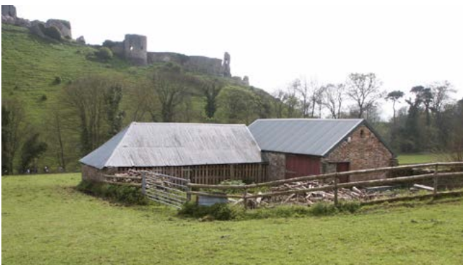
A small outfarm consisting of a three-bay shelter shed and a small building for storage for fodder. Photo © Bob Edwards
