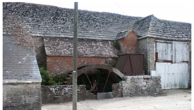
Unusually for this area, this large, 18th-century barn has a water wheel to power threshing machinery. Photo © Bob Edwards
