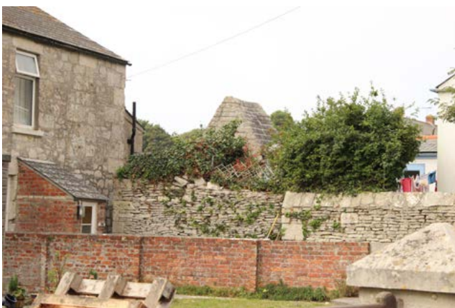
A glimpse towards an outbuilding behind a village house of uncertain function but possibly originating as an agricultural building. Photo © Bob Edwards
