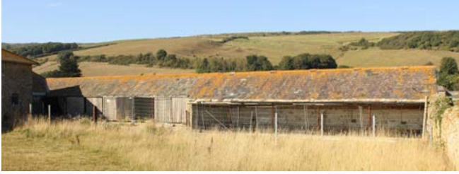
A ten-bay open-fronted shelter shed of late 19th-century date, illustrating the requirement for farms to manage large numbers of fat stock. The use of slate for the roof and cast iron for the posts to the front are typical of this date. Photo © Bob Edwards
