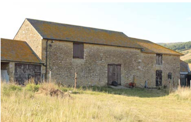
A 19th-century barn and attached stable forming part of an L-plan farmstead outside of the village of Abbotsbury. The barn is probably partly floored, as suggested by the large pitching door at upper level. The asymmetrical position of the threshing bay suggests that unthreshed corn was pitched into the left-hand side of the barn, the straw being taken straight to the cattle yard. Cart sheds are attached to the left and the stable to the right also has a hayloft. Photo © Bob Edwards
