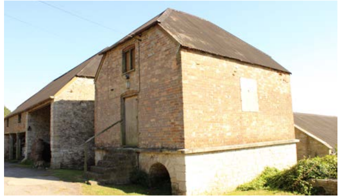
The buildings on this farm illustrate the scale and requirements of the large, arable-based farms that developed in this area. To the left is an early to mid-19th-century granary and cart shed range. The later and taller bay to the right may have housed larger equipment such as a traction engine. To the right is an early 19th-century, brick granary built on stone arches, typical of Dorset generally where timber-framed staddle granaries are rare. Photo © Bob Edwards
