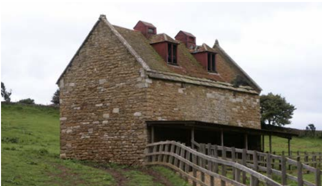
Buildings for sheep are of exceptional rarity. Farms on the southern chalk downs made use of barns and walled farmyards for shearing, and the very low eaves height to some shelter sheds suggests that they were constructed for sheep rather than cattle. Notably, the roof is of solid thatch, a rare survival nationally. Photo © Bob Edwards
