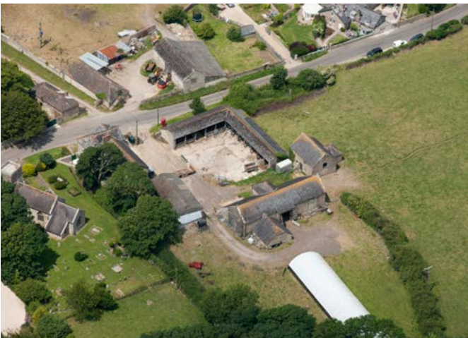
The Manor Farm in Swyre is a dispersed multi-yard plan farmstead with two main yard areas either side of the village street. The main yard is across the road from the farmhouse and has a five-bay barn (a very late example of a threshing barn which is internally dated 1888), a small stable (set back to the right of the yard) and an L-plan range of open-fronted shelter sheds for cattle closing two sides of the yard. Across the street is a yard with a second barn and a cart shed with granary over – steps against the gable wall give access to the granary. Photo © Historic England 29076/016
