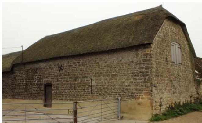
Many barns in this area have double doors to one side only with a small door opposite for obtaining a through draft for winnowing. The end-bay was lofted and probably served a different function from the three bays of the barn, defined by the ventilation slits and door to the threshing bay. Photo © Bob Edwards
