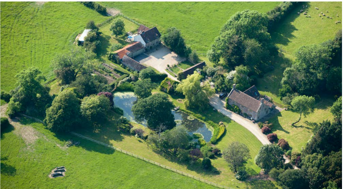
A loose courtyard farmstead group with buildings to three sides of the yard with the 17th-century farmhouse set away and some distance from the working area. Note the large farm pond. Photo © Historic England 29107/036
