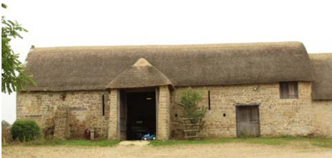
Barns are slightly more common on farmsteads in the Powerstock Vale than in the Marshwood Vale. This 16th- or 17th-century barn on a high-status farmstead combines a threshing barn with a stable and its hay loft to the right. Blocked doors to the left suggest that there was once more animal housing within the building whilst external steps to the gable gave access to a granary. To the rear there is later horse engine house. Photo © Bob Edwards
