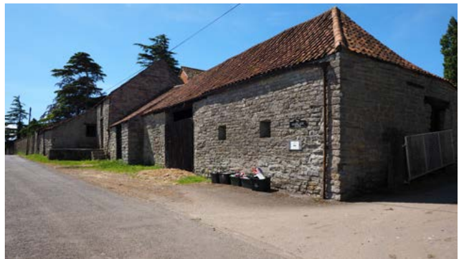
This early to mid-19th-century range at Upper Godney comprises a threshing barn, a hay barn and a cow house with a later lean-to addition. Note the steps to the churn stand, for loading milk onto lorries; these were commonly introduced from the 1920s. Photo © Eric Berry
