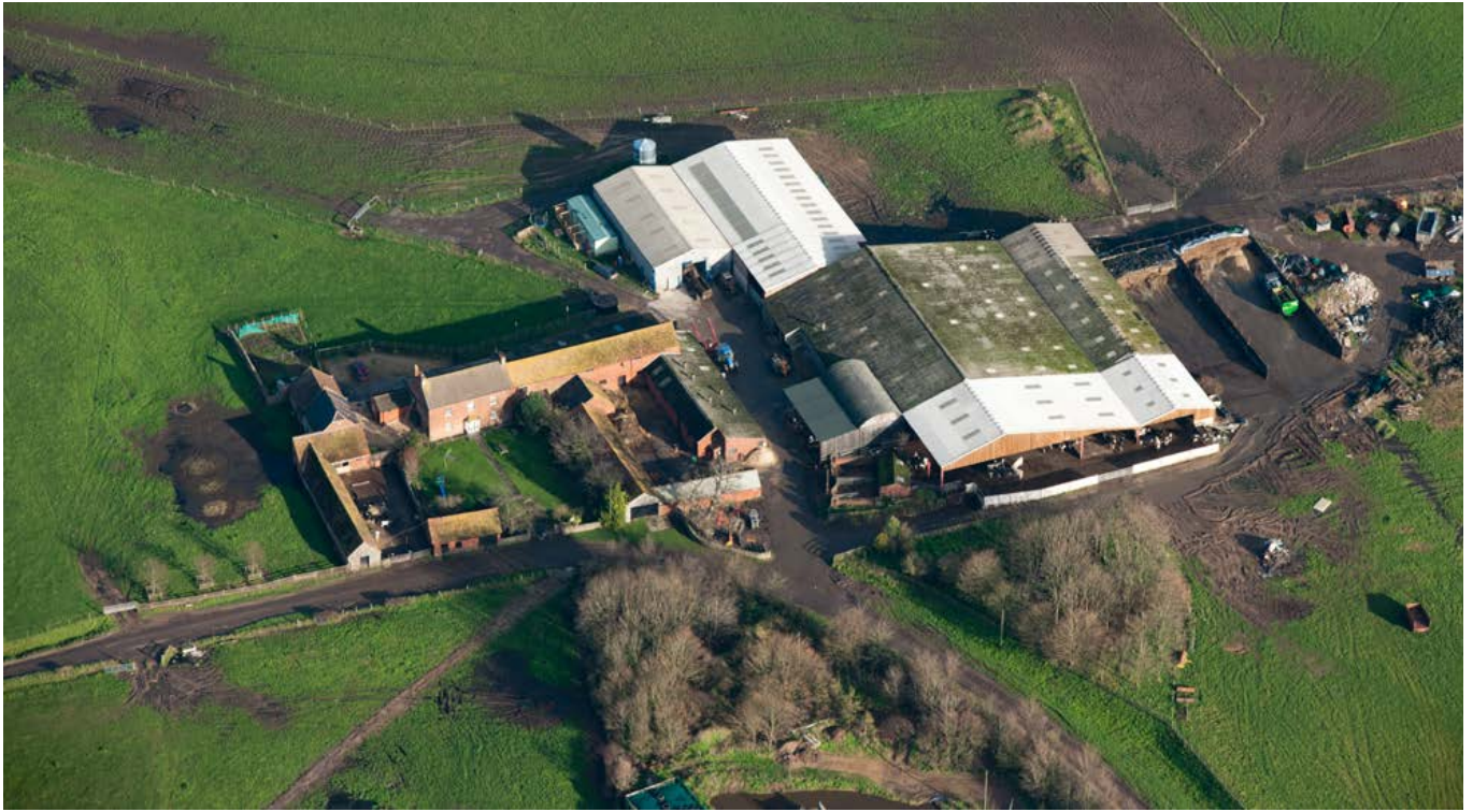
Detail of a regular multi-yard farmstead built in the early to mid-19th century, with a south-facing farmhouse and linked yards. It is subdivided from left into a stock yard with shelter sheds and a dairy, the house with its garden and cart shed facing the road, and a barn and stockyard to the right. Photo © Historic England 27896/014
