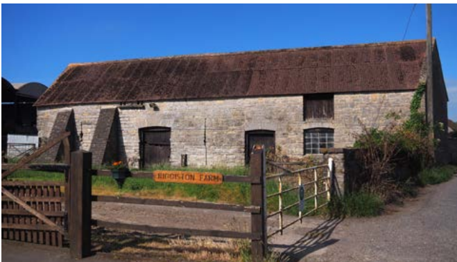
An early 19th-century combination barn at Buscott. Note the doveholes above the door to the threshing floor, with its winnowing door; to the right is a hay loft over stables. Photo © Eric Berry
