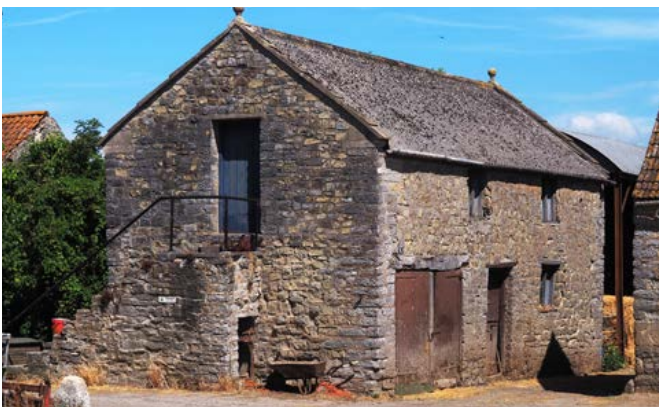
A rare-surviving, late 18th-century combined stables, cart shed and first-floor granary with its external steps. This is near Meare; note the dog kennel below the granary steps and the ball finials to the stone-coped gable ends. Photo © Eric Berry
