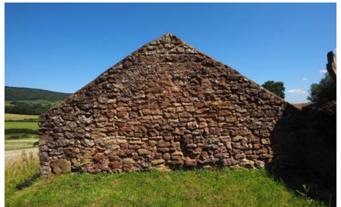
The outline of an earlier building in a stone-walled gable. Photo © Eric Berry
