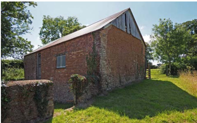
Many buildings that made use of cob, as here, at Holcombe, were built on tall plinths and have been partly or wholly rebuilt in brick or concrete block. Photo © Eric Berry
