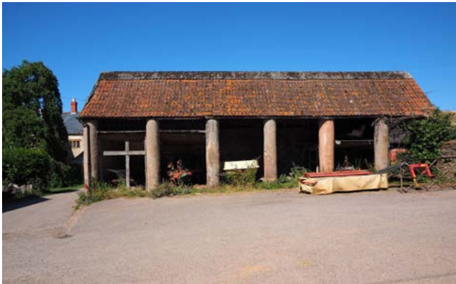
Open-fronted lincays for cattle, with slight timbers to a hay loft above housing for fatstock, are a feature of this area. Photo © Eric Berry
