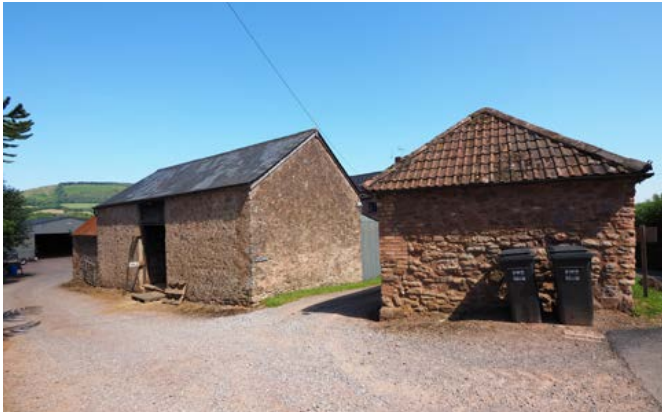
A small, three-bay, early 19th-century barn (at Walcombe) devoted to storing and processing the corn crop, typical of smaller farmsteads and as built up to the mid-19th century. Photo © Eric Berry
