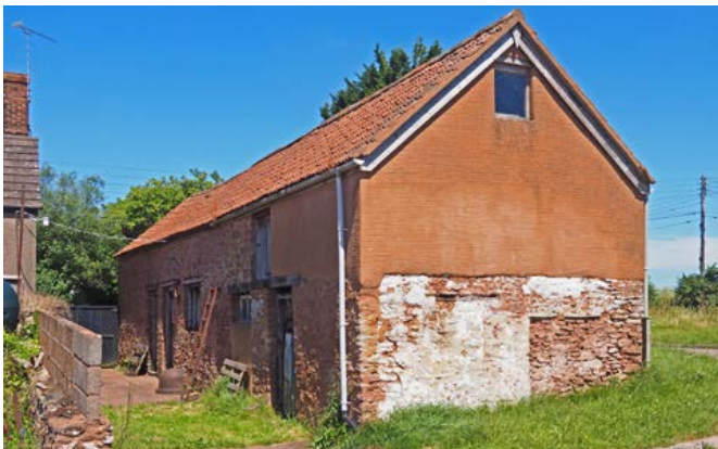
Another part-cob and stone building at Halse. Photo © Eric Berry
