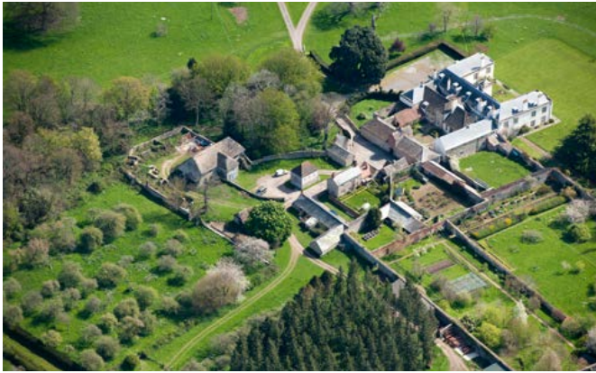
The home farm at Fairfield House (see map on page 7) has developed with several farmyards on a piecemeal basis. To the left is a 17th-century barn with a porch; to its right is a pyramidal-roofed granary and close to the house are late 18th-century stables with a dovecote. Cattle yards were added in the early to mid-19th century. Photo © Historic England 27975/038
