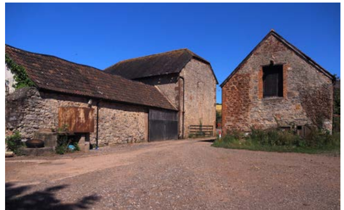
A typical feature of this area is the relationship of single-storey cattle housing to taller combination barns (to the left) and stables with hay lofts (to the right). Photo © Eric Berry
