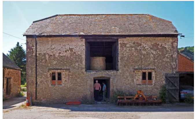
A range of c 1840 near Watchet, with open-fronted cart sheds attached to a threshing barn with an internal loft. Photo © Eric Berry
