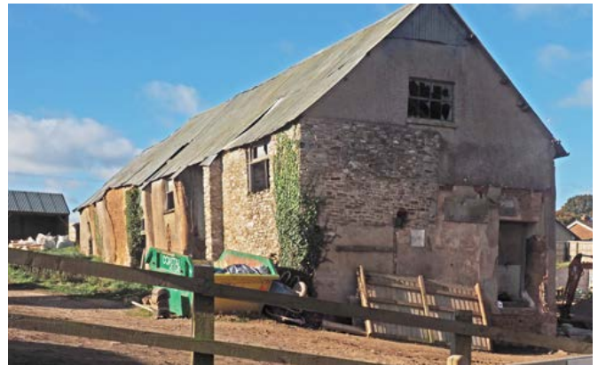
A 17th- to 18th-century threshing barn built of cob, with two threshing floors and partly rebuilt in stone rubble. Photo © Eric Berry
