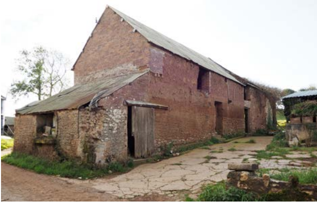
Cob was also used for large barns, cattle housing and stable ranges, as here, and has often been repaired and rebuilt in places with stone rubble and, from the later 19th century, in brick. Photo © Eric Berry
