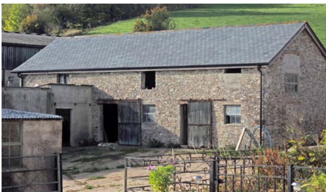
The large size of arable-based farms, as they developed in some parts of the area in the early to mid-19th century, called for large stable ranges. This range was reroofed and converted to a cow house for dairy cattle, with metal-framed windows, in the mid-20th century. Photo © Eric Berry
