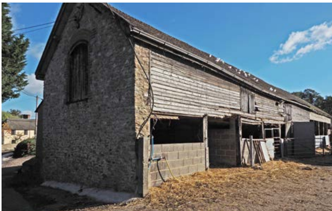
A large, mid- to late 19th-century linhay for cattle, with later weatherboarding applied to its originally open-fronted hay lofts. Photo © Eric Berry
