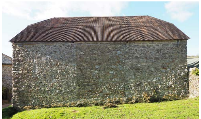
Many threshing barns were converted into housing for dairy cattle from the late 19th century. Note how the central threshing bay has been infilled in stone rubble walling. Photo © Eric Berry
