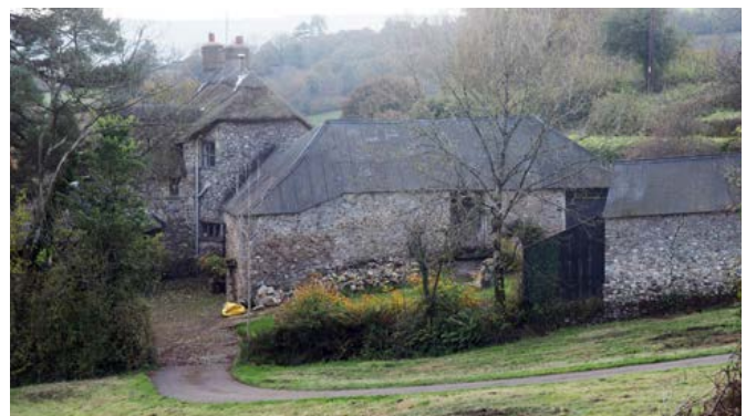
An 18th-century bank barn is attached to one end of this 17th-century farmhouse. This is an early type of bank barn, built into the slope and with a door to a stable or cow house to the lower gable end. Photo © Eric Berry
