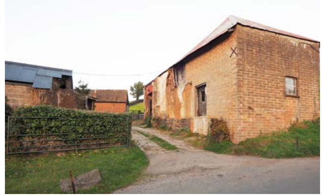
An early 19th-century combination barn with an integral stable in the foreground, partly rebuilt in concrete block. Photo © Eric Berry
