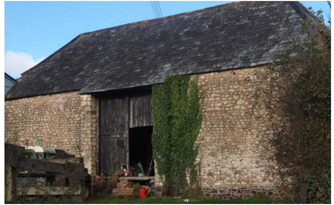
A late 18th- or early 19th-century threshing barn, its hipped roof replaced by Welsh slates. Note the raised threshing floor, which would have been boarded. Photo © Eric Berry
