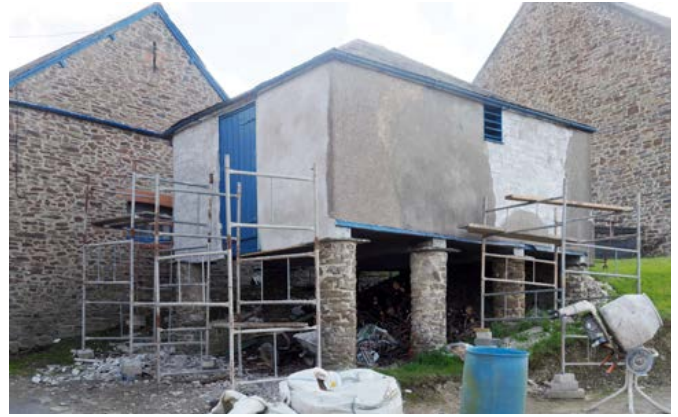
A late 18th- or early 19th-century granary, raised on piers to keep the grain dry and out of the reach of vermin. Photo © Peter Child
