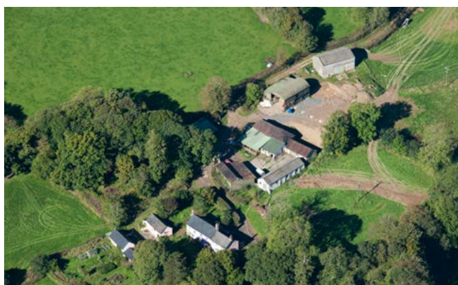
A farmstead to the north of Stoodleigh Beacon, sited at the junction of routeways for driving stock to moorland. The site has retained its dispersed multi-yard plan form, and the farmhouse, which includes a cider house, is a 17th-century remodelling of an earlier house. Photo © Historic England 27856/009
