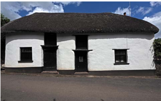
17th-century stables and shippon (cow house) in cob and thatch at Sampford Courtenay. Photo © Eric Berry
