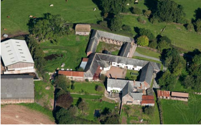
High-status farms developed as large courtyard layouts. Bury Barton (see p 2), which developed within the Taw valley, developed as a barton from the late 14th century. The medieval hall house is attached to an early 19th-century cider house and store, and has a service entrance to the farmyard flanked by a barn (with a horse engine house of c 1850 in the angle of the yard), stables and linhays dating from the 16th century. Linhays face into the early to mid-19th-century outer yard, and there is a 15th-century chapel to top left of the image. Photo © Historic England 27857/041
