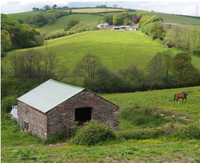
Field barns were built in the late 18th and 19th centuries, often built into hillsides, as here, in the South Hams. Photo © Eric Berry
