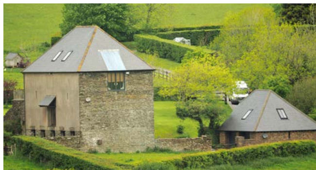
Another early to mid-19th-century combination barn with a canopied door to the threshing floor above housing for cattle. Photo © Eric Berry
