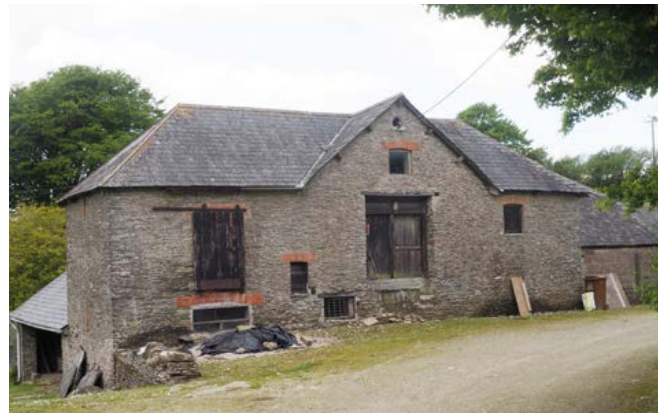
High levels of investment in the early and mid-19th century have resulted in the rebuilding of many earlier farmsteads, and of a wide variety of combination barns. This late 19th-century bank barn has a sliding door (as introduced from the 1850s) and a small entry for the drive shaft of a mobile steam engine. Photo © Eric Berry
