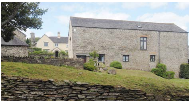
An early 19th-century combination barn, now in residential use, with a winnowing door for creating a through-draught for winnowing threshed corn over the threshing floor. Photo © Eric Berry
