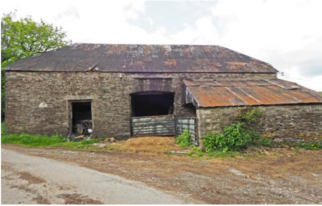
An early 19th-century combination barn with a shippon (cow house) to the left and a cart shed in a lean-to to the right. Corrugated iron has been in common use since the later 19th century. Photo © Eric Berry
