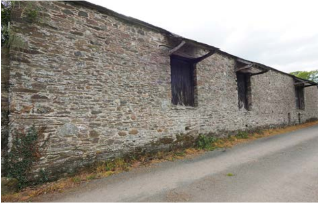
Three canopied doors indicate the exceptionally large scale of this barn with its three threshing floors. Photo © Eric Berry
