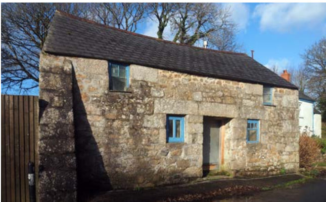
Vellanewson: a late 18th-century to early 19th-century mill next to a small farmstead. Without the evidence of the wheel this is virtually indistinguishable in scale, details and use of materials from similar farm buildings (although those are otherwise rare, especially this early, in Carnmenellis). Photo © E Berry.
