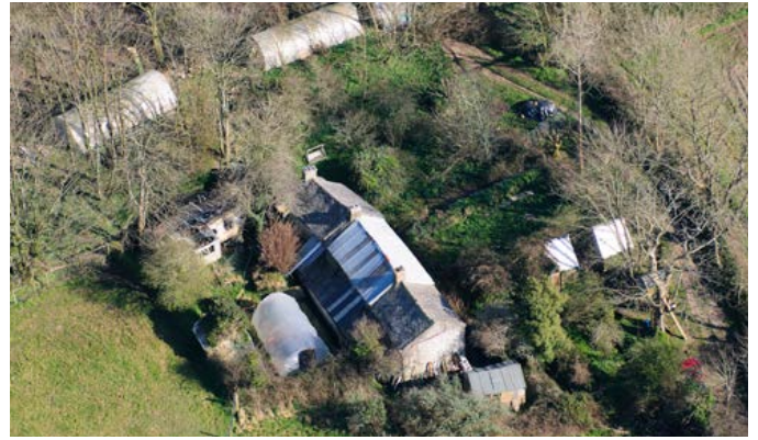
Smallholding, Polcrebo Moors. Small 17th-century or earlier house, extended and remodelled in 18th century and in 1836 (datestone); a row of cottages formed out of house and farm-building unit. Photo © Historic Environment, Cornwall Council, 2009; F90-116.
