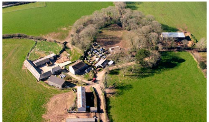
Tregear, Crowan parish. A medieval farm (a tre settlement – one of the primary settlement types in the Cornish landscape), not only takes its name from the adjacent round, but exploits it for a yard. The present farmhouse and improved courtyard developed over the 19th century – the earlier buildings were within and on the ramparts of the round itself. Photo © Historic Environment, Cornwall Council, 2009; F90-053.
