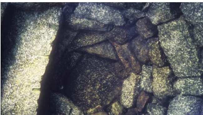
Helland: goose house, interior showing corbelled roof construction. Photo © E Berry.
