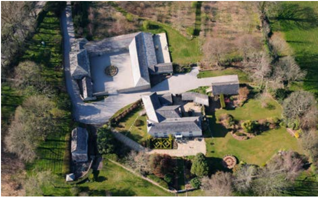
Medieval manorial site at Cosawes. Improved regular courtyard with good 18th-century farmhouse and cottage plus farm buildings including barn, shippens and good example of a horse-engine house, all with scantle slate roofs. Photo © Historic Environment, Cornwall Council, 2009; F90-019.
