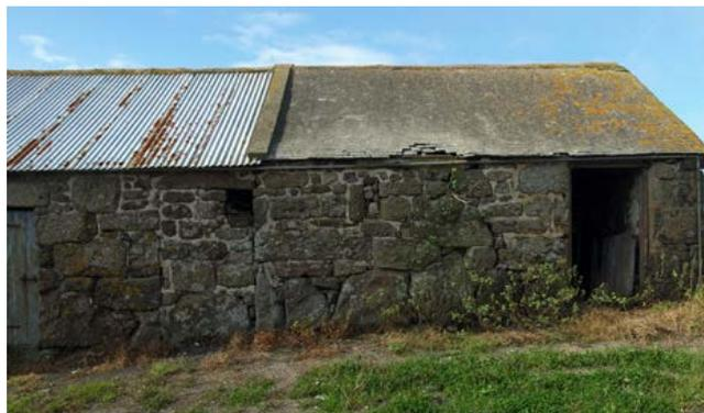
Slate roofs are the norm – traditionally wet-laid (i.e. set in mortar), with diminished courses getting smaller as they rise to the ridge, and typically lime or cement washed as added protection. Photo © Eric Berry.
