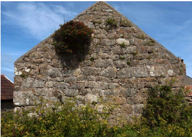
St Agnes, Middle Town. Granite is the predominant traditional building material; squared and coursed stonework, even on farm buildings, show a degree of traditional local craftsmanship. Photo © Eric Berry.
