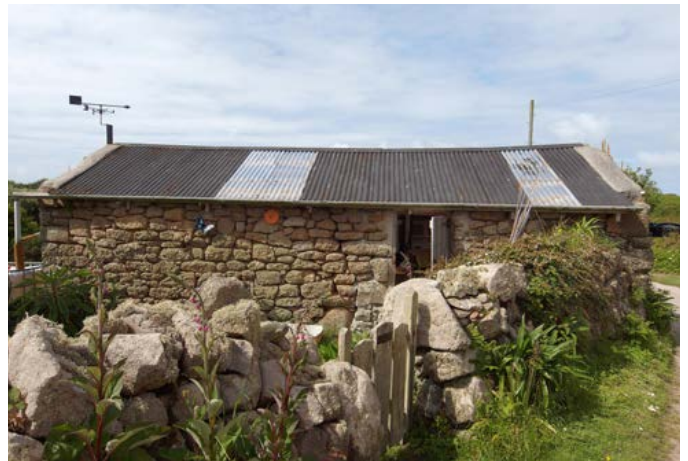
Granite is also found as simple, rough dry stone walling, and more random rough-coursed construction. Photo © Eric Berry.
