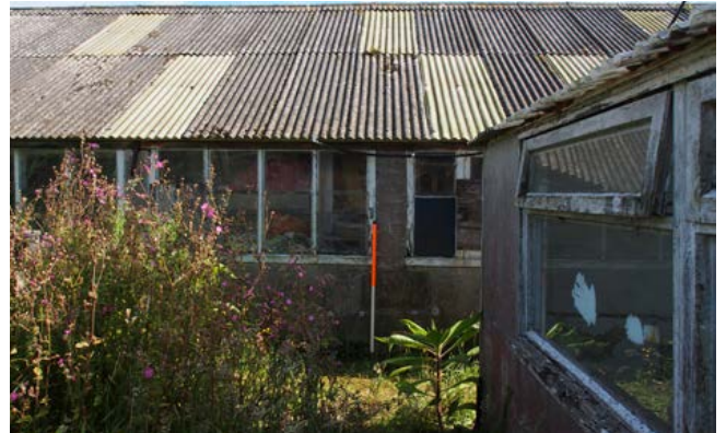
St Mary's. Early 20th-century glasshouses – concrete blocks, timber windows and corrugated roofing; an increasingly rare building type replaced by modern metal-framed structures, or by plastic polytunnels. Photo © Eric Berry
