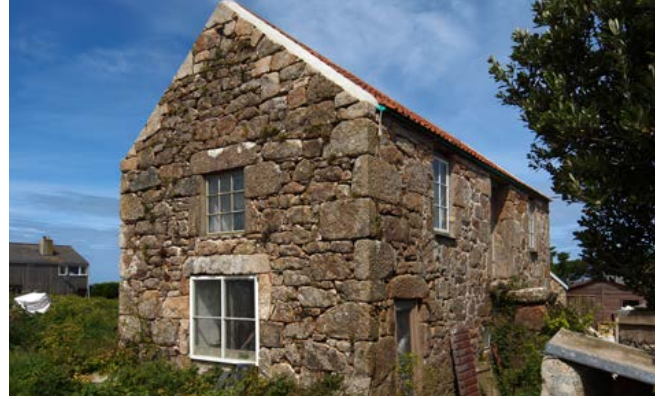
Two-storey combination barn, with external steps to upper floor threshing areas; not in domestic use, but much re-use of old windows; note the pantile roof. Photo © Eric Berry.
