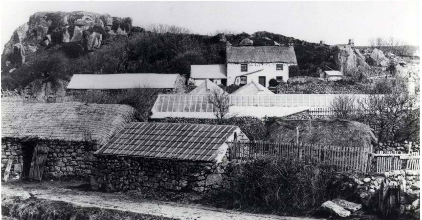
Ennor Castle. Building types and building materials – thatch, pantile, glasshouse, and dry stone walls... (all gone...). Photo from the Gibson Archive.
