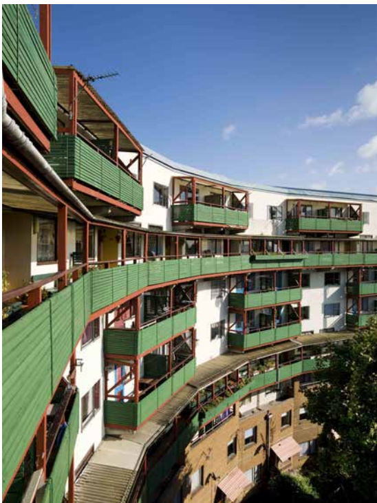
Figure 31: Byker Estate, Tyne and Wear, Ralph Erskine, 1970-82. Photograph by James O. Davies; © English Heritage.
