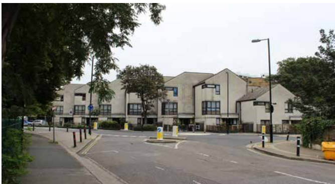
Figure 26: Wiltshire Road / Sisulu Close (completed 1992, main job architect Abe Hayeem). (SP004003).
