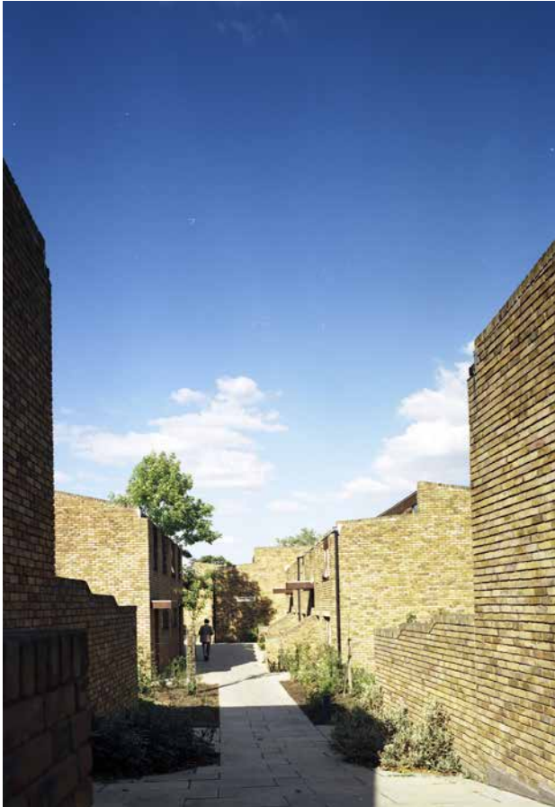
Figure 21: Pedestrian walkway at the Cressingham Gardens estate. Photograph kindly provided by Charles Attwood.
