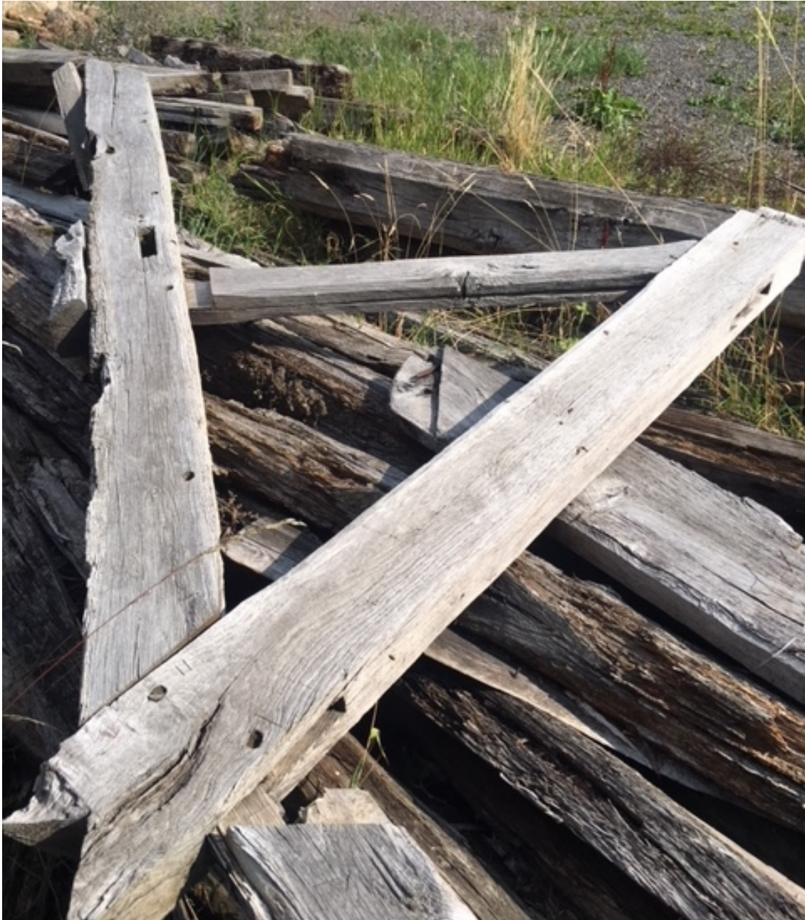
Figure 7: Pile of ex situ timbers, possibly discarded original trusses (Alison Arnold)
