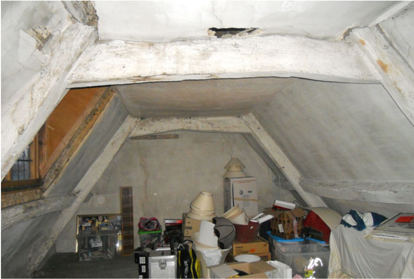
Figure 3: View of the east-range roof, looking south (photograph Martin Bridge)
