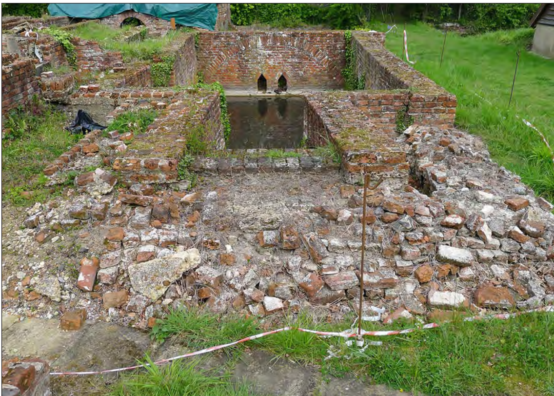
Figure 19 – The Large Cellar from the south with the block of brickwork wrapping around the south stair. Note the possible joint to the lower left, the second joint is obscured by the buff block (Jonathan Kewley 26/04/2017 © Historic England)
