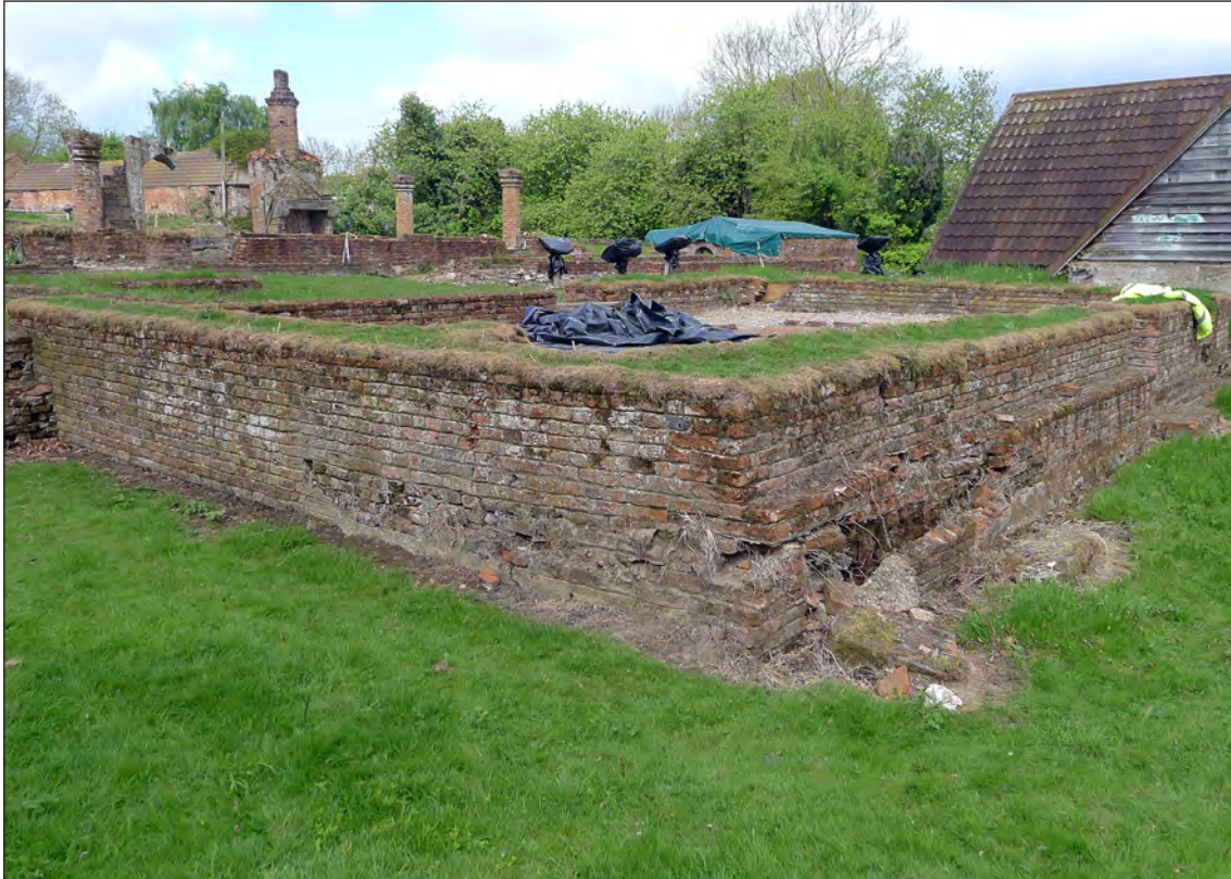
Figure 45 – A general view of the Kitchen from the south-east. Note the slightly decayed early work in the base of the wall to the left of the near corner and the late work spalling away from earlier work to the right (Jonathan Kewley 26/4/2017 © Historic England)
