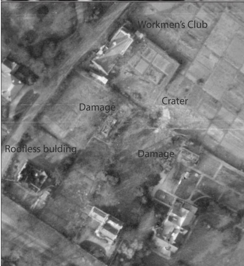
Figure 91 – Workmen's Club and surrounding area after air raid. Detail of RAF/106G/UK/1339 RV 6265 29-MAR-1946. Historic England Archive (RAF Photography)
