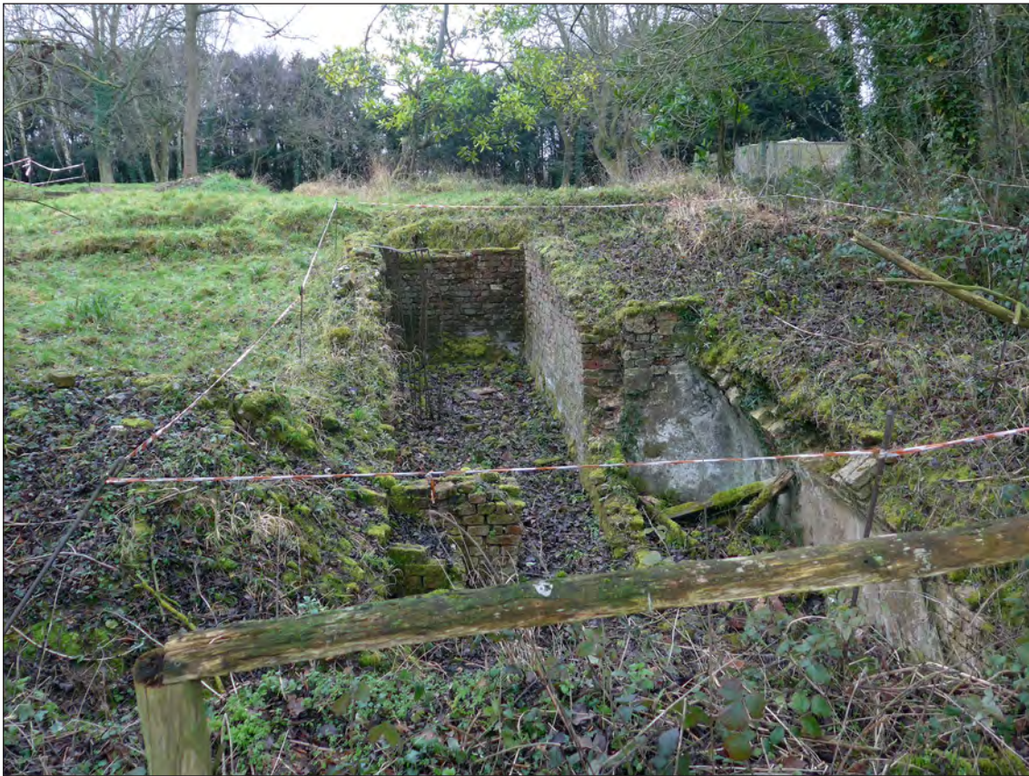
Figure 59 – The cellar of Scadbury Park Mansion from the north, note the vault spring to the right, English bond brickwork is visible in places (Magnus Alexander 14/2/2018 © Historic England)
