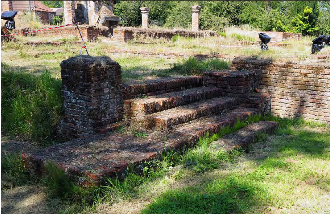
Figure 46 – Steps to the south of the Kitchen (Magnus Alexander 11/8/2020 © Historic England)
