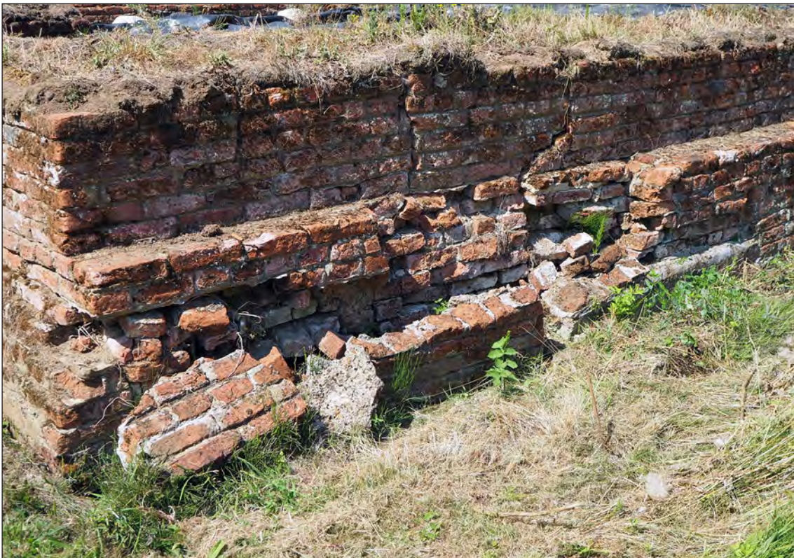
Figure 49 – The south end of the east wall of the Kitchen, from the south-east, showing the late skin falling away from the probably early core (Magnus Alexander 11/8/2020 © Historic England)
