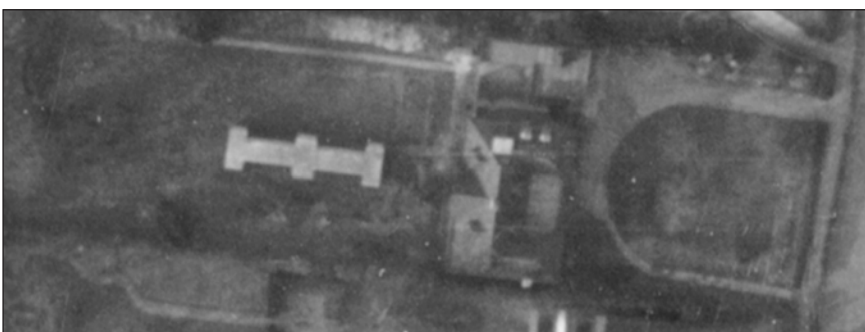
Figure 81 – War-time building in the garden of Chesham House. Detail of RAF/106G/UK/1339 RV 6309 29-MAR-1946. Historic England Archive (RAF Photography)
