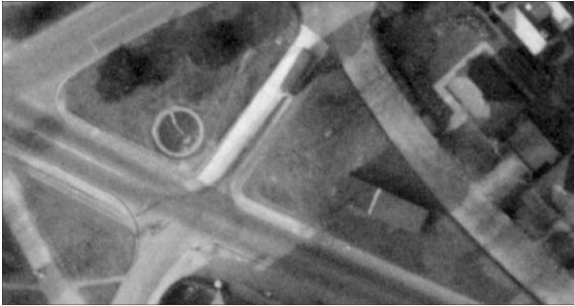
Figure 85 – Rectangular air raid shelter (right) and circular Emergency Water Supply (left) on Royal Parade. Detail of RAF/106G/LA/1339 RV 6264 29-MAR-1946. Historic England Archive (RAF Photography)
