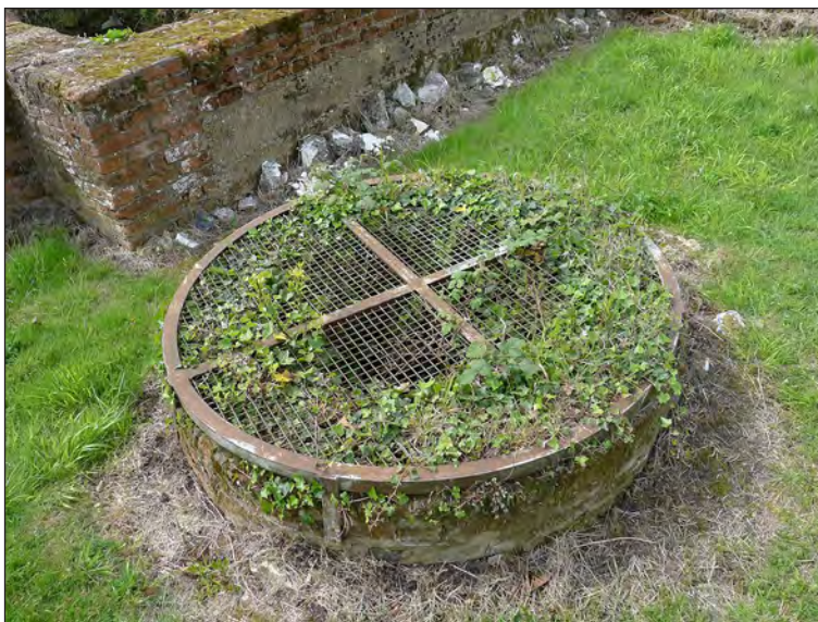
Figure 16 – The north well from the north-east. The late north wall of the Large Cellar can be seen in the background, note the use of concrete (Jonathan Kewley 26/04/2017 © Historic England)
