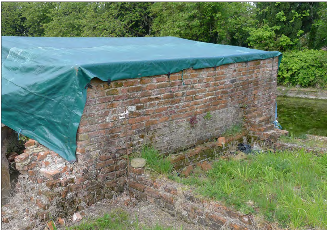
Figure 21 – The east wall of the Undercroft showing the late work above and the stepped-out section below (Jonathan Kewley 26/04/2017 © Historic England)
