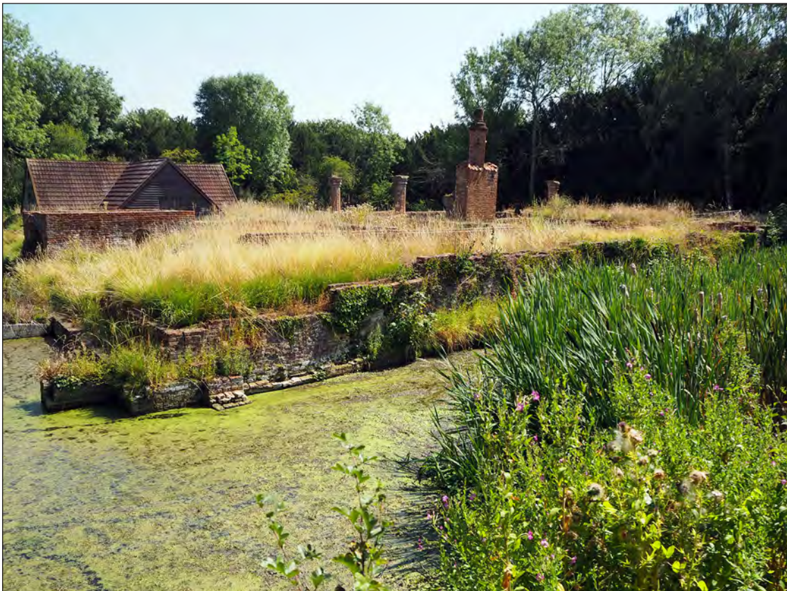
Figure 34 – A general view of the moat island from the north-west, with the west moat wall from the north-east corner to the bridge abutment (Magnus Alexander 11/8/2020 © Historic England)
