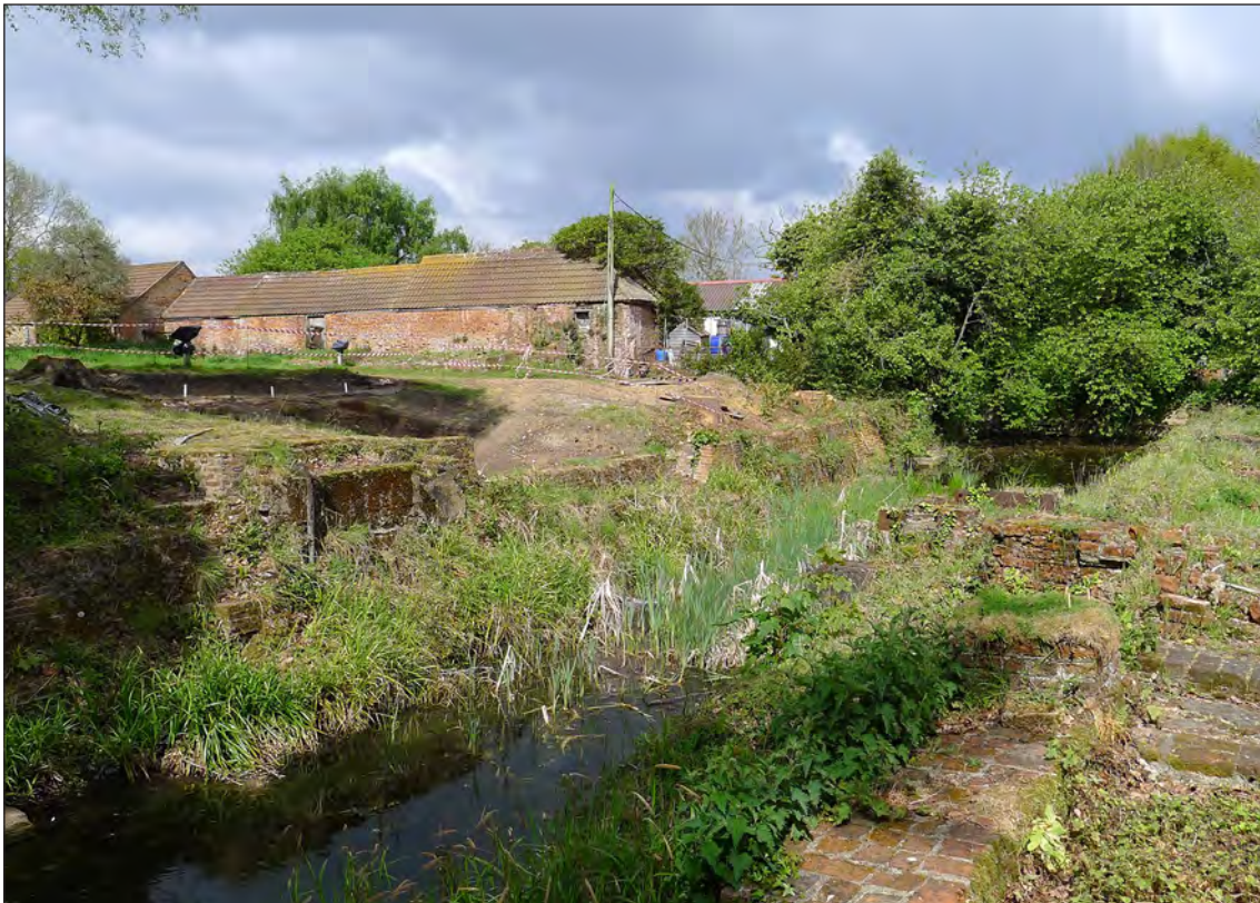
Figure 54 – A general view along the west moat arm looking north (Jonathan Kewley 26/4/2017 © Historic England)
