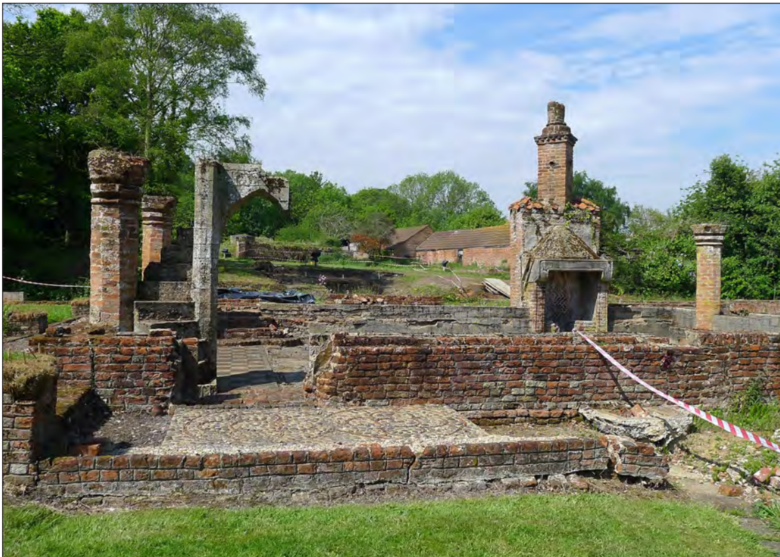
Figure 39 – A general view of the Hall area from the south-east. Three of the four brick columns, the concrete stair and the fireplace are visible, the decorative pavement in front of the south-east door (middle foreground) is typical of the other late decorative pavements laid by the Marsham-Townshends seen elsewhere (Jonathan Kewley 11/5/2017 © Historic England)
