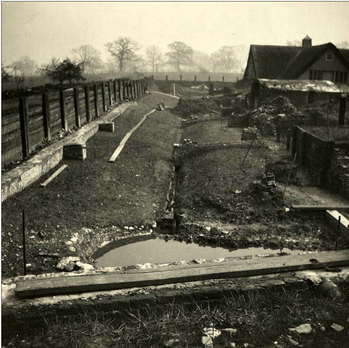
Figure 10 – An example of one of the excavation photographs of the 1920s showing the north moat arm from the west (BHC, 1080/2/1/17)
