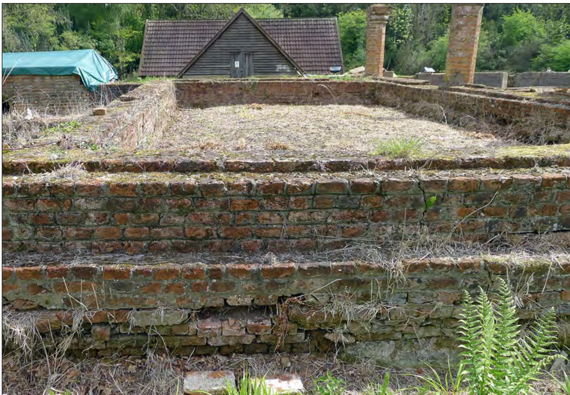
Figure 30 – The Parlour from outside the north-west corner looking east. Note the decaying English bond at the base of the wall with some late concrete to the right (Jonathan Kewley 26/4/2017 © Historic England)
