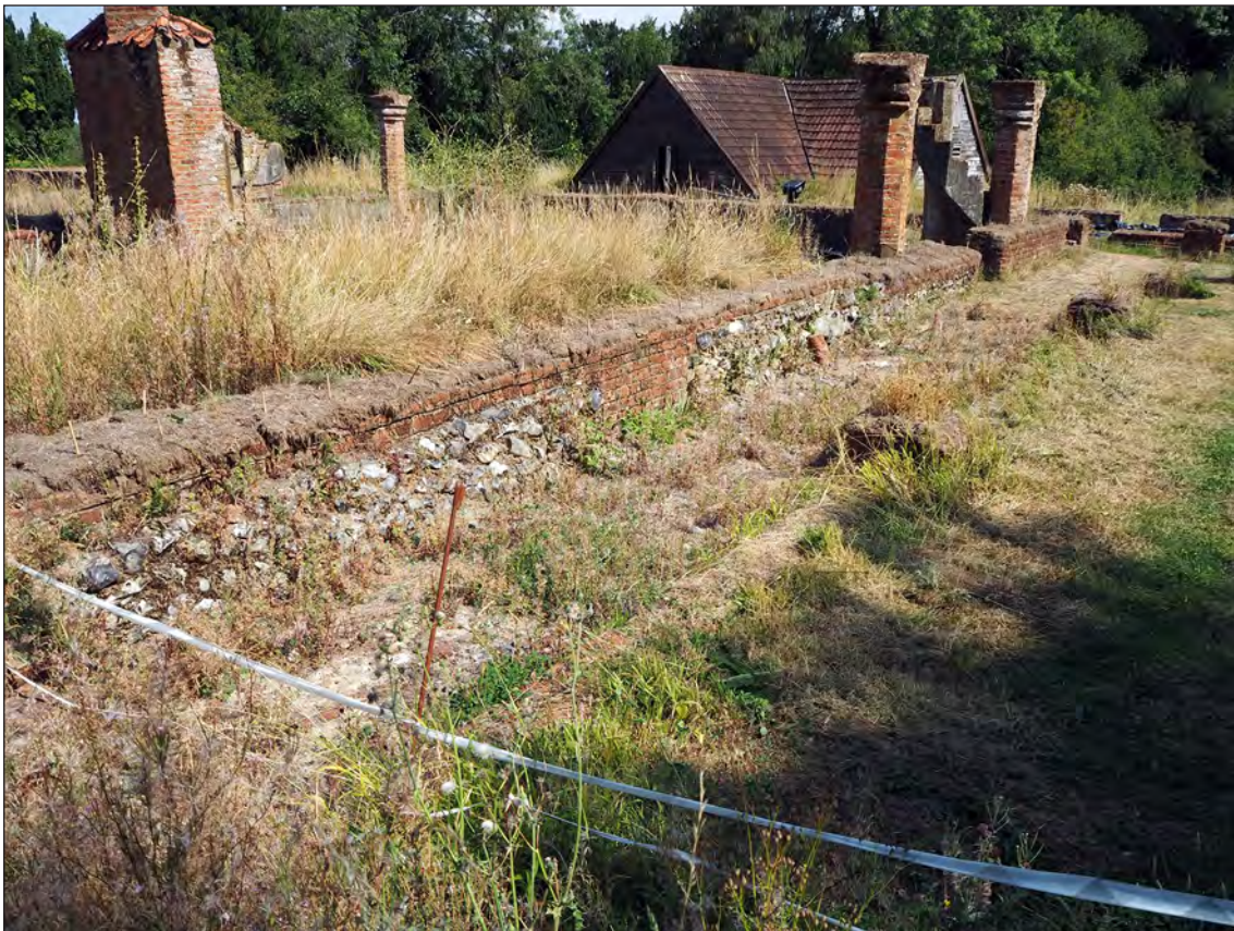
Figure 37 – General view of the flint wall from the WSW, the bricked up section, possibly an entrance, can be seen in the centre of the image (Magnus Alexander 11/8/2020 © Historic England)
