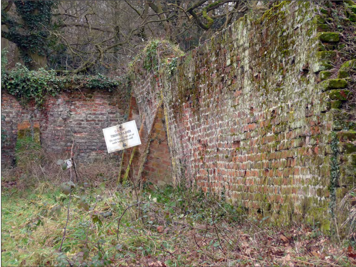
Figure 60 – The western corner of the walled garden from the ENE showing the buttresses supporting the leaning north wall (Magnus Alexander, 14/2/2018, © Historic England)
