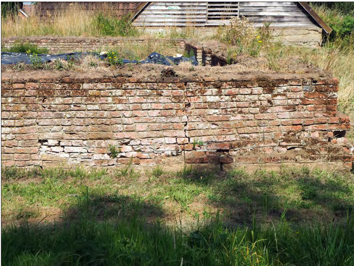
Figure 50 – The east end of the south Kitchen Wall, note the presence of English bond towards the base (Magnus Alexander 11/8/2020 © Historic England)
