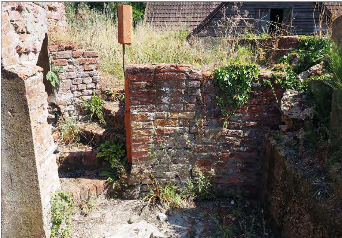
Figure 26 – The east of the Undercroft ‘area’, the area of concrete and rubble to the right is the location of one of the steps noted on the Gotch and Saunders survey plan (Magnus Alexander 11/8/2020 © Historic England)
