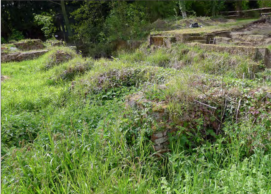
Figure 35 – The west moat wall from the north, despite being rather overgrown, four of the internal buttresses are visible with the bridge abutments on the island (left) and opposite (above right of centre) visible beyond (Jonathan Kewley 26/4/2017 © Historic England)
