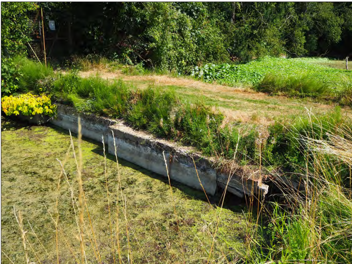
Figure 14 – The Causeway from the south-west, note the cast concrete reinforcement and the brick to the right (Magnus Alexander 11/08/2020 © Historic England)
